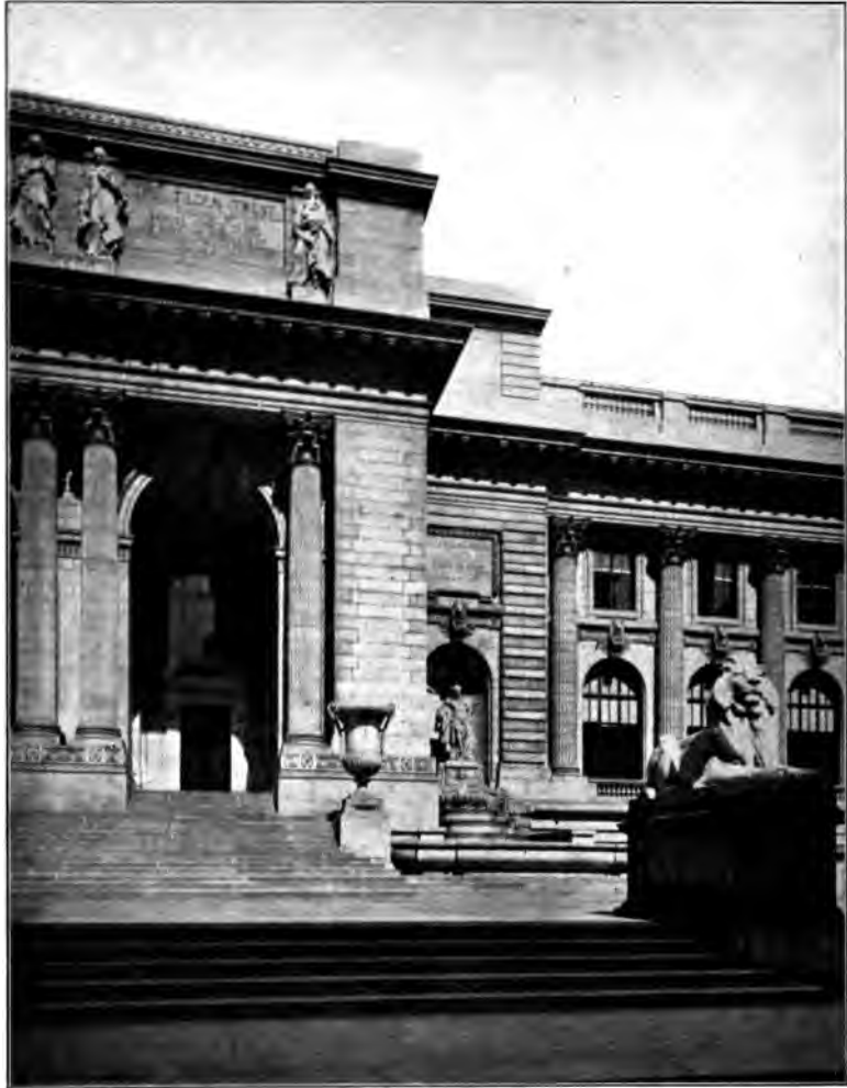
PART OF MAIN FACADE
