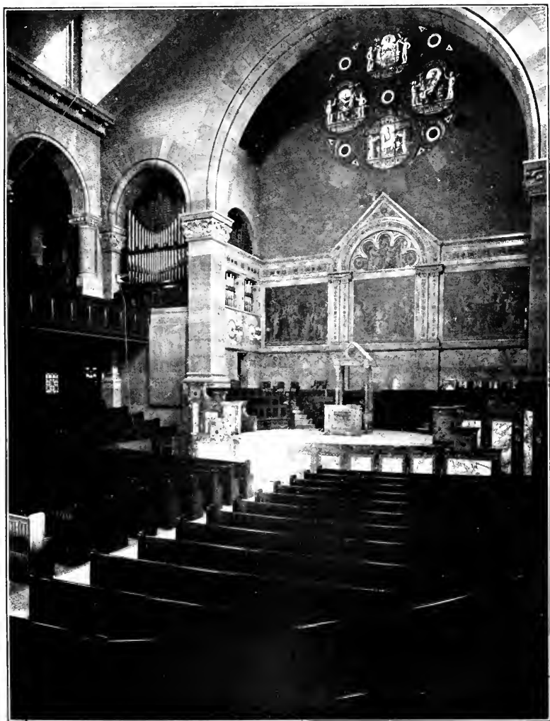
INTERIOR OF ALEXANDER HALL By courtesy of the American Architect
