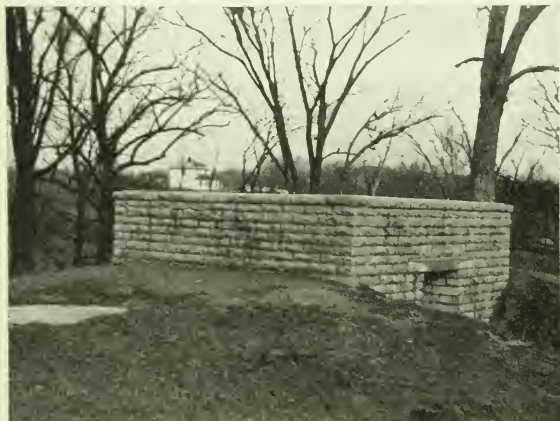
W. H. HARRISON'S VAULT, 1897.
