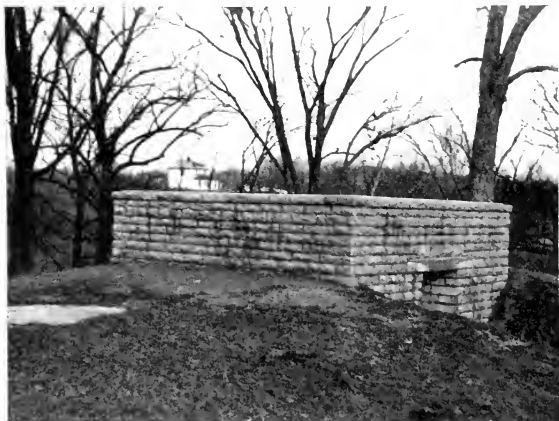
W. H. HARRISON'S VAULT, 1897.
