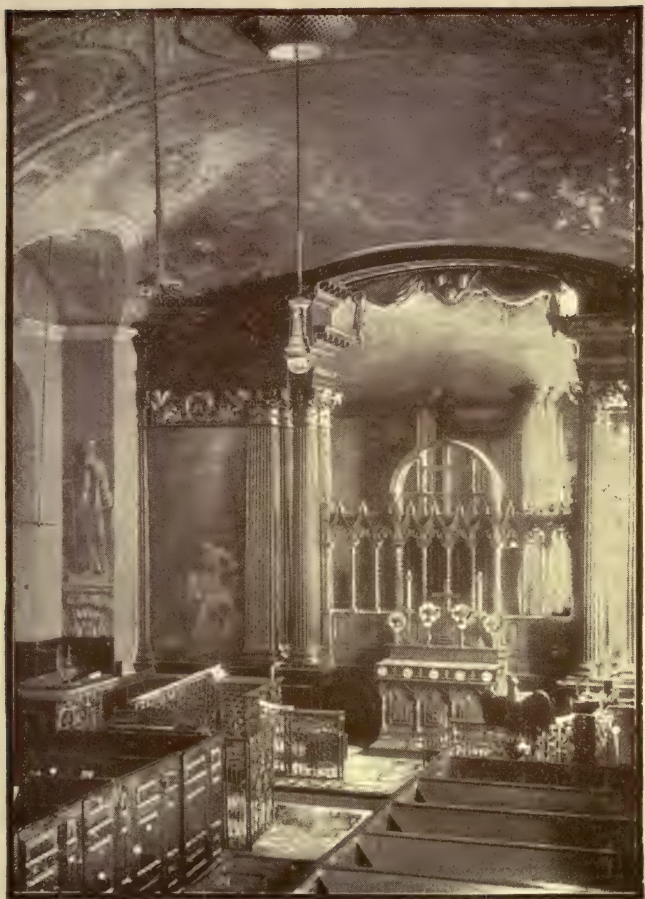
Interior of Whitchurch Church
