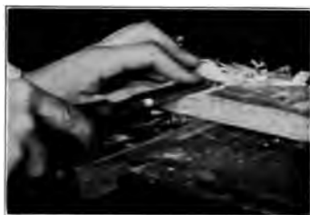
Fig. 71. Chiseling Out a Dado (Second Step).
