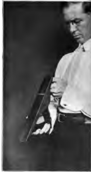
Fig. 102. Sighting Along the Sole of Jack-Plane.
