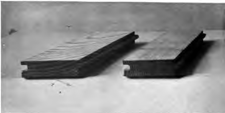
Fig. 55. Slash-Grain and Comb-Grain Flooring.
