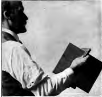
Fig. 203. Using the Try-Square.
