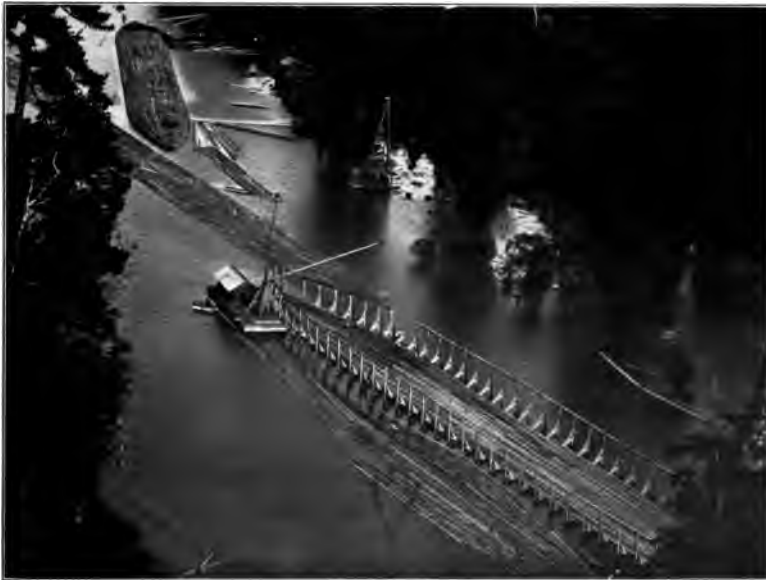
Fig. 30. Giant Raft. In the background is a completed raft; in the foreground a cradle in which a raft is being built.
