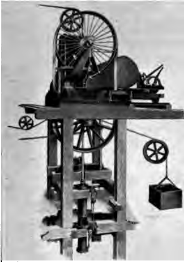
Fig. 35. Double-Cutting Telescopic Band-Mill. Mill in raised position for large log.
