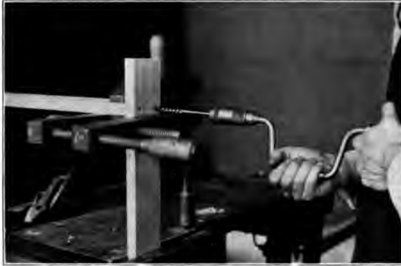
Fig. 247. Thru Boring for a Butt Joint.
