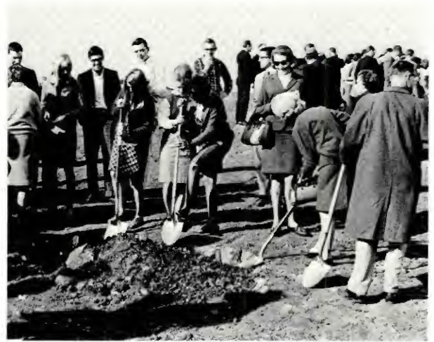
The groundbreaking – November 15, 1966
