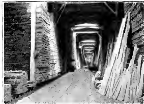
INTERIOR OAK FLOORING WAREHOUSE, M. B. FARRIN LUMBER COMPANY.
