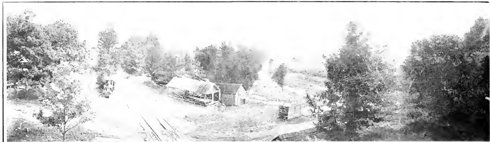
PICTURESQUE AND WELL-ORDERED BAND SAWMILL PLANT OF R. E. WOOD LUMBER COMPANY.
