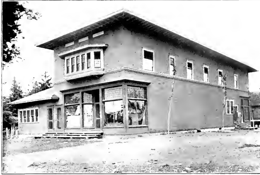
STORE AND OFFICE BUILDING AT HACKLEY.
