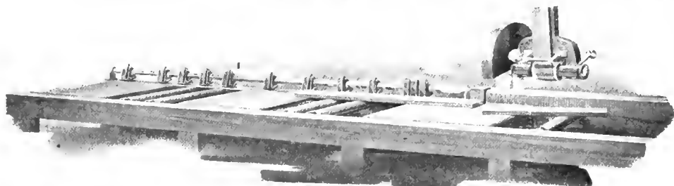
AUTOMATIC SWING SAW GAUGE
