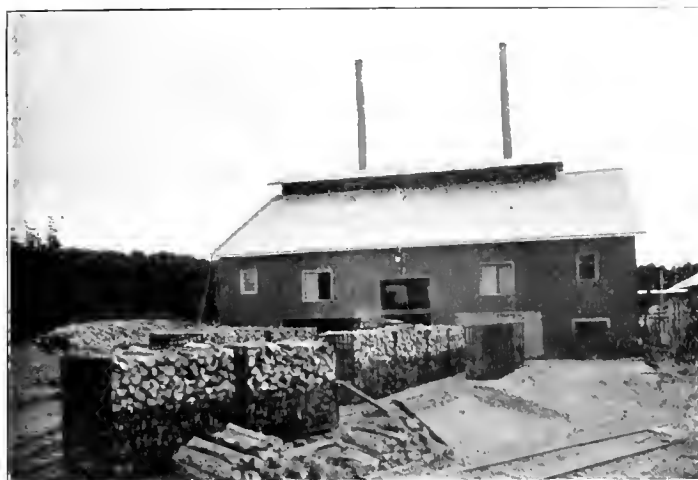
RETORT HOUSE OF CHEMICAL PLANT AT HACKLEY.
