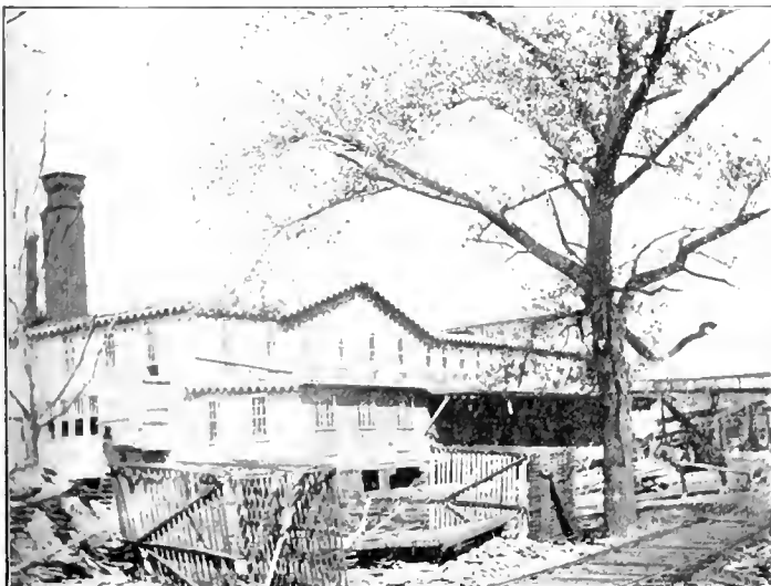
PLANT, PREWITT-SPURR MANUFACTURING COMPANY
