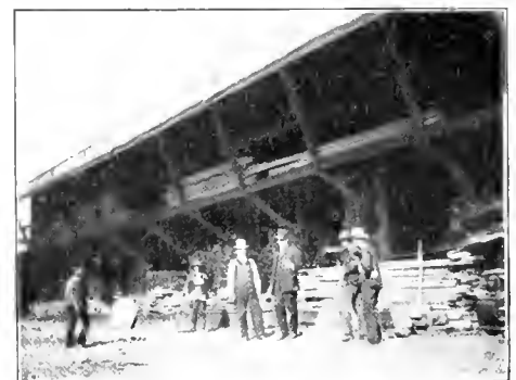
LUMBER SHEDS, STANDARD BOX & LUMBER COMPANY.
