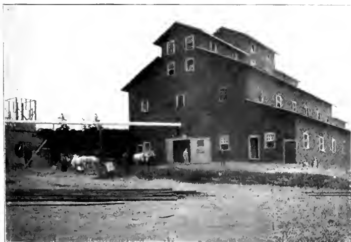
STILL HOUSE OF THE CHEMICAL PLANT.
