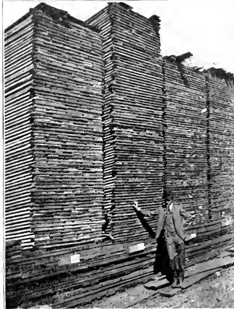
SCENE IN YARD, PREWITT-SPURR MANUFACTURING COMPANY.
