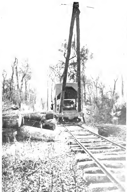
PULLING SKIDDER THROUGH
