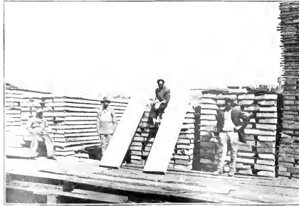
A COUPLE OF BIG ONES AND SOME MORE IN PILE
