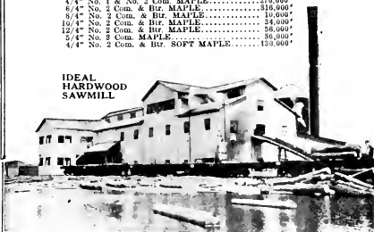
Are putting in pile every month two and one-half million feet of choicest Northern Michigan Hardwoods
