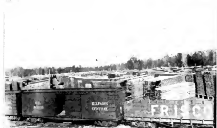
Corner of Proctor Lumber Yard
