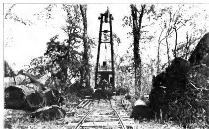
Loader Ready for Work
