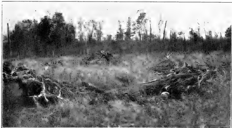
The Results of a Well Placed Charge of Dynamite.
