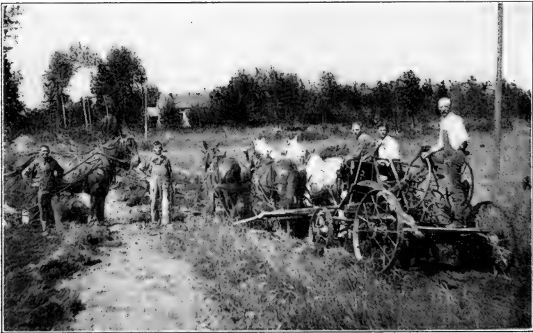
Road Making by the Use of the Grader.
