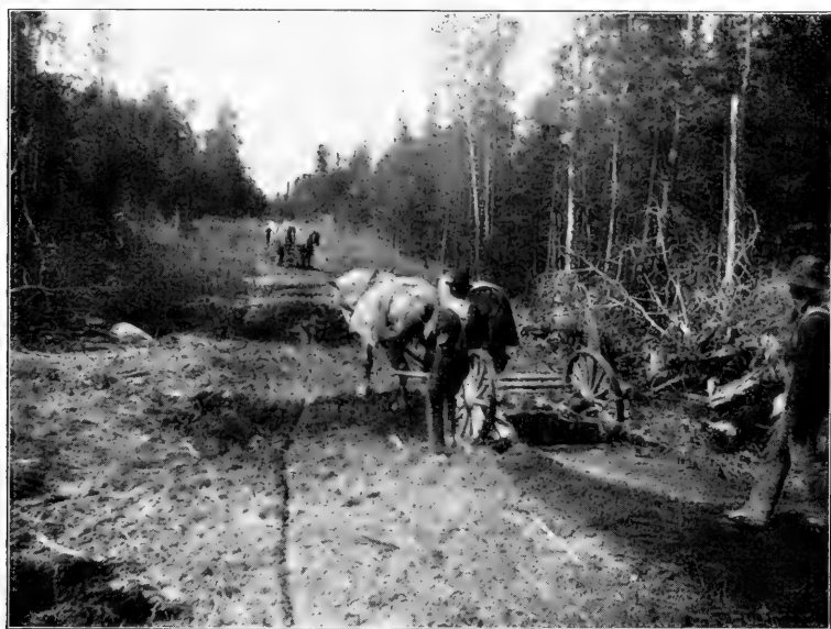
Road Making Through the Virgin Forest.
