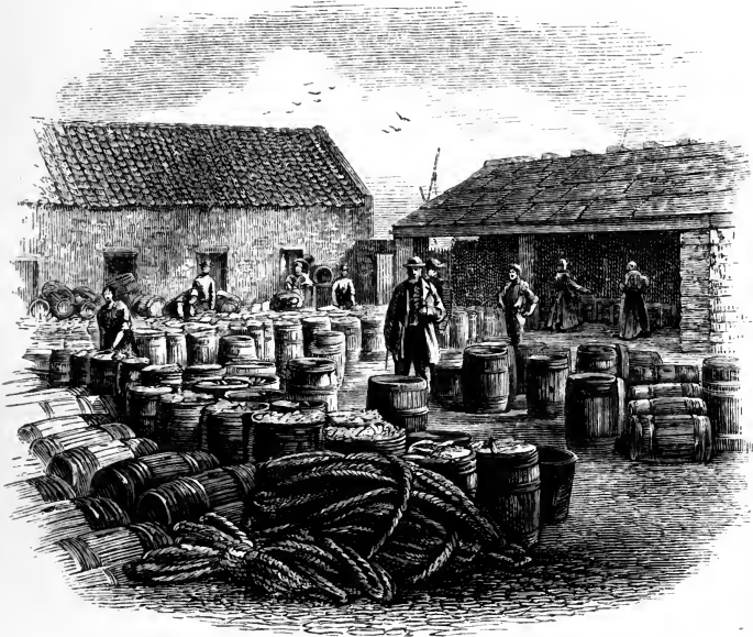
VIEW OF A CURING YARD.
