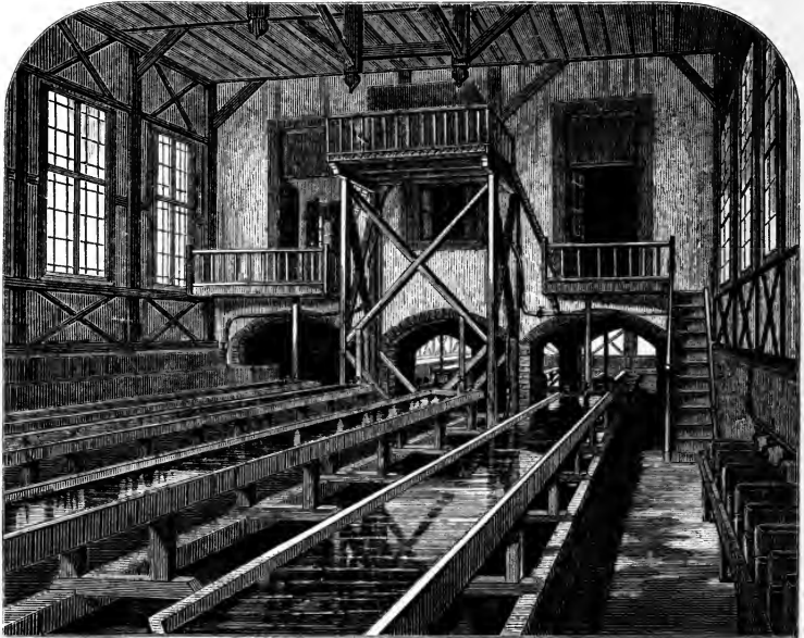
GUTTERS FOR HATCHING PURPOSES.
