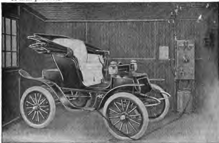
FIG. 4,089.—View showing Studebaker electric in home garage connected to rectifier charging outfit. The subject of rectifiers has been treated at such length in Guide No. 6, that no further explanation is here necessary.
