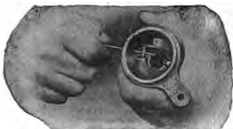
FIG. 3,999.—Filing slot for cleaning platinum contacts of Connecticut magneto interrupter. The cup holding the interrupter or primary circuit breaker may be withdrawn from its housing. The slot serves as a guide for a small flat file for cleaning and squaring the contact points. By means of an adjustable gauge furnished with the magneto, the correct opening of the contact points may be determined. The interrupter is provided with a single roller bearing against the cam pins, thus insuring accurate timing at any speed and unaffected by centrifugal force. The advance lever can be connected at either side of the magneto as the interrupter housing is reversible. The cams are renewable by a half turn with a screw driver.
