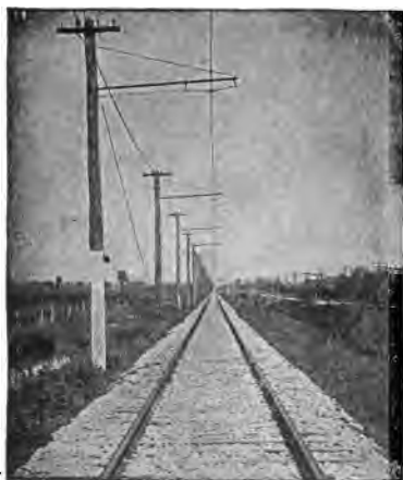
FIGS. 3,499 and 3,500.—Overhead construction on the Indianapolis & Louisville 1,200 volt line. The line throughout is of the single bracket construction on tangents, as shown in fig. 3,499 and of the span type at curves, as in fig. 3,500. The poles are spaced 90 ft. apart on tangents and 60 ft. on curves. A single No. 0000 trolley wire of grooved section is used, and is held in alignment by 8 in. four screw clamps reinforced with soldered strain guys every half mile. Lightning arresters are installed every 1,000 ft., and are tapped alternately to the trolley and feeder. Telephones have been installed throughout the system, and jack boxes are attached to the poles at all sidings and at half-mile intervals.
