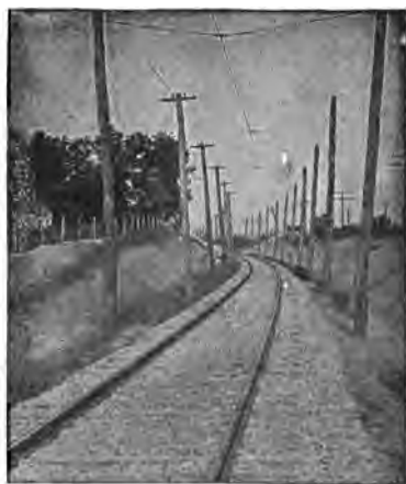
FIGS. 3,499 and 3,500.—Overhead construction on the Indianapolis & Louisville 1,200 volt line. The line throughout is of the single bracket construction on tangents, as shown in fig. 3,499 and of the span type at curves, as in fig. 3,500. The poles are spaced 90 ft. apart on tangents and 60 ft. on curves. A single No. 0000 trolley wire of grooved section is used, and is held in alignment by 8 in. four screw clamps reinforced with soldered strain guys every half mile. Lightning arresters are installed every 1,000 ft., and are tapped alternately to the trolley and feeder. Telephones have been installed throughout the system, and jack boxes are attached to the poles at all sidings and at half-mile intervals.
