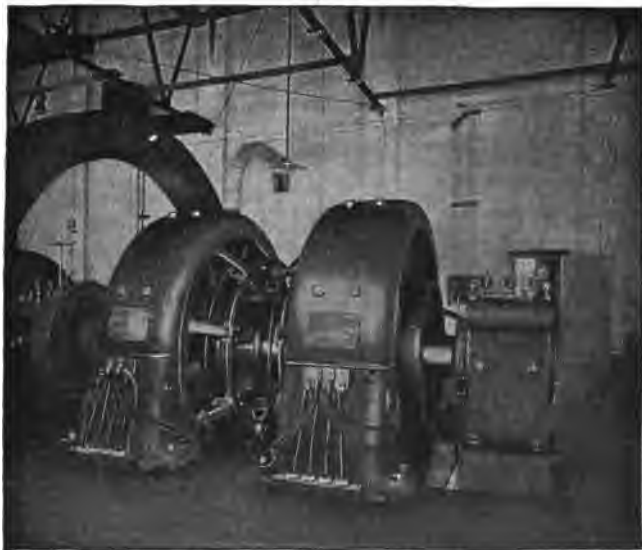
FIG. 3,497. —Interior of power station at Scottsburg (Indianapolis & Louisville line), showing direct connected two stage units. The two dynamotors as shown are mounted on the extended shaft of each engine (there being two sets), and the armatures are connected in series to give 1,200 volts. The fields are connected in series on the ground sides. The switchboard consists of two dynamo panels, two feeder panels, and two exciter panels. The switches are all of the knife pattern. The control is of the automatic Sprague-General Electric parallel unit type. The commutating switch used on these equipments is located on the car platform beside the master controller for convenience in operation. The operating mechanism of the contactors is similar to those used on standard 600 volt equipments, the only difference being that additional insulation is used. The protective devices are similar to those on standard 600 volt equipment with the exception of additional blowout capacity in the main fuse bores. As is usual on 1,200 volt equipments, a dynamotor is provided to supply 600 volts for the auxiliary circuits, including the secondary control, lighting and compressor circuits.
