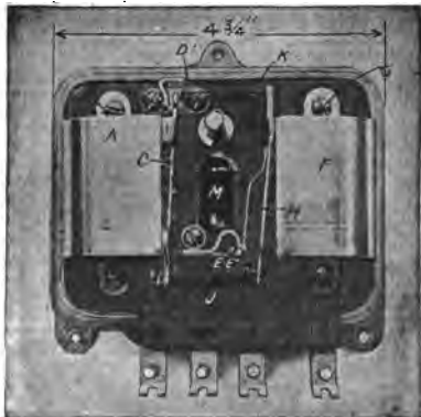
FIG. 4,054. —Ward Leonard automatic controller for automatically regulating the charging of the battery. When the car speed becomes approximately seven miles per hour, the dynamo armature will give a voltage sufficient to charge the batteries. The circuit between the dynamo and the batteries is normally open, but when the voltage of the dynamo becomes proper for charging, the coil A on the magnet core B, magnetizes the core sufficiently to attract the arm C. This arm moves toward the core B and thus two spark proof points D D' are brought together, establishing the circuit between the battery and the dynamo, and the dynamo begins to charge the batteries. In a dynamo the dynamo voltage increases with the speed unless a method of controlling it be adopted. The dynamo should charge at about seven miles per hour, but it is desirable that when the car runs at a much higher speed, as 15 to 60 miles per hour, the dynamo voltage shall not increase. If allowed to increase, such an excessive dynamo voltage would tend to cause sparking at the brushes, excess current and consequent trouble at the commutator and excessive wear and heating of the bearings. It would also cause an excessive amount of current to flow through the battery. To prevent this, the strength of the dynamo field, and consequently the output of the dynamo, is made dependent on the touching of the two points E E'. The coil F on the magnet core G carries the armature current, and if this current become a certain amount (usually in practice 10 amperes) the core becomes sufficiently magnetized to attract the finger H. This separates the contacts B E' and a resistance M is inserted in the field circuit, weakening it. This causes the amperes flowing through the battery to decrease. When the current decreases to a predetermined amount (say 9 amperes), the coil F does not magnetize the core G enough to overcome the pull of the spring J. The spring J pulls together the points E E', the full field strength is restored and the current tends to increase. Under operating conditions, the finger H vibrates so rapidly as to keep the current constant. As a result the dynamo will never charge above a predetermined amount (10 amperes), no matter how high the speed of the car, but at all speeds greater than a predetermined speed (about 15 miles per hour in practice), the dynamo will charge at a varying rate, which has a maximum of 10 amperes and a minimum of 9 amperes. In case the engine speed become so low that the dynamo cannot charge the battery, the magnetism caused by the coil A is weakened so that the spring K pulls the contacts D D' apart. Thus the circuit between the dynamo and battery is opened when the dynamo speed is too low for the dynamo to charge. The auxiliary series coil L on core B acts to insure the perfect demagnetization of the core B on reversal of current.
