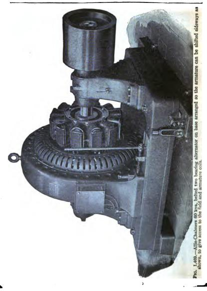
On alternators of the fly wheel type the spider rim is made of sufficient weight to obtain full fly wheel effect, thus making a separate fly wheel unnecessary.
