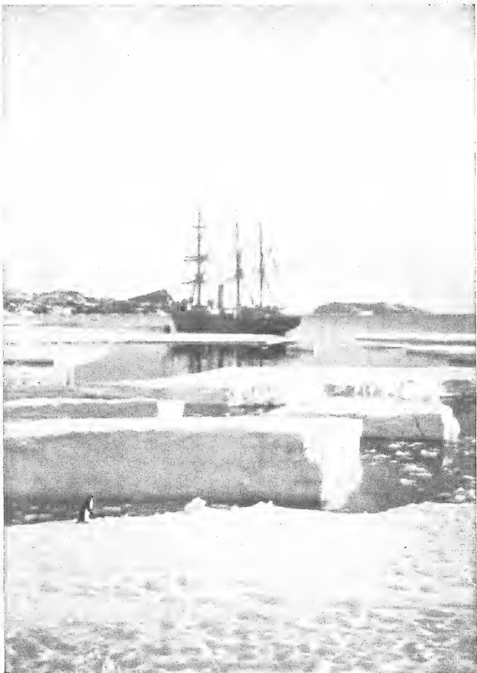
THE LANDING-PLACE WHARF BROKEN UP
