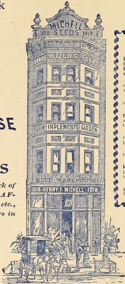
Our new building, erected last summer. Depth, 190 feet.
