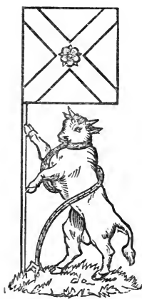
No. 419.—SUPPORTER OF THE NEVILLE SHIELD. From Butleigh Court, Somerset.
