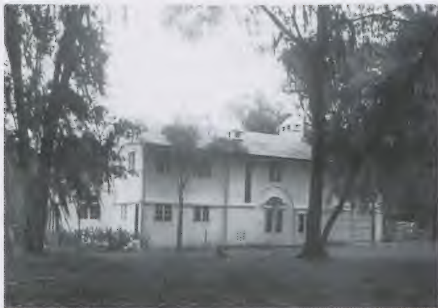
Figure 6. H.P. Traub's residence, Mira Flores, at Orlando, Florida.
