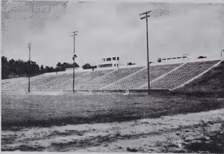
Burlington High School Stadium
