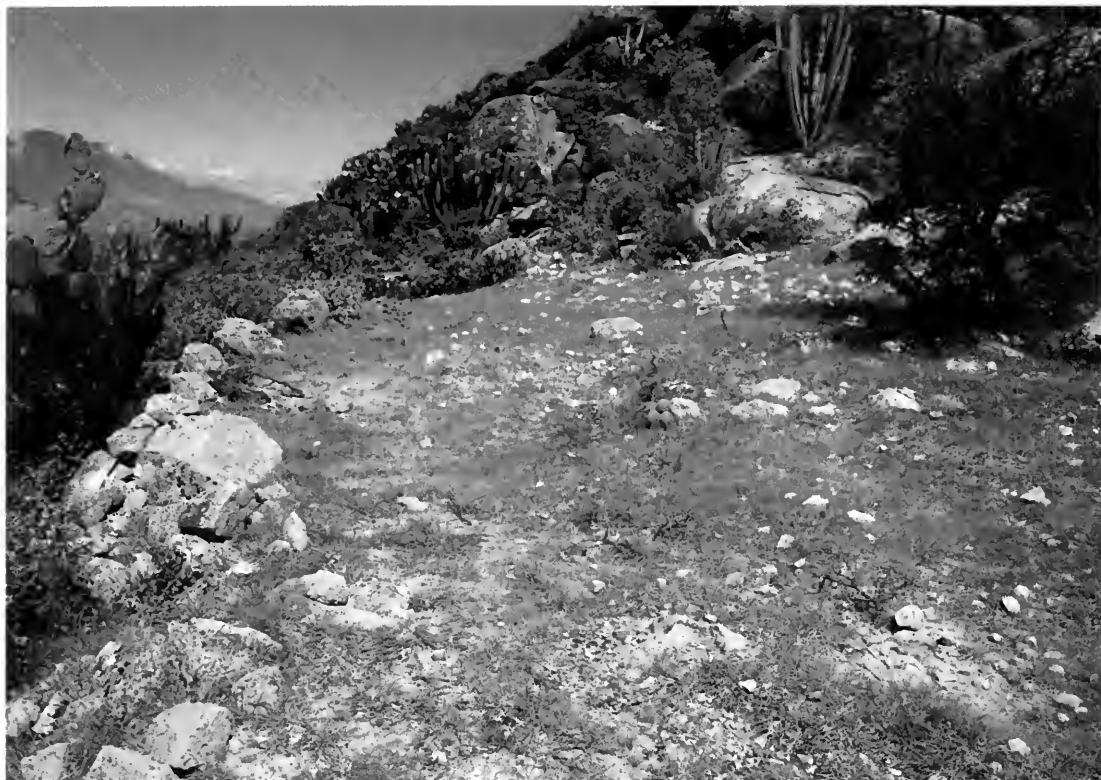
FIG. 3.10. Terrace 276 with house foundation at the Mitla Fortress.
