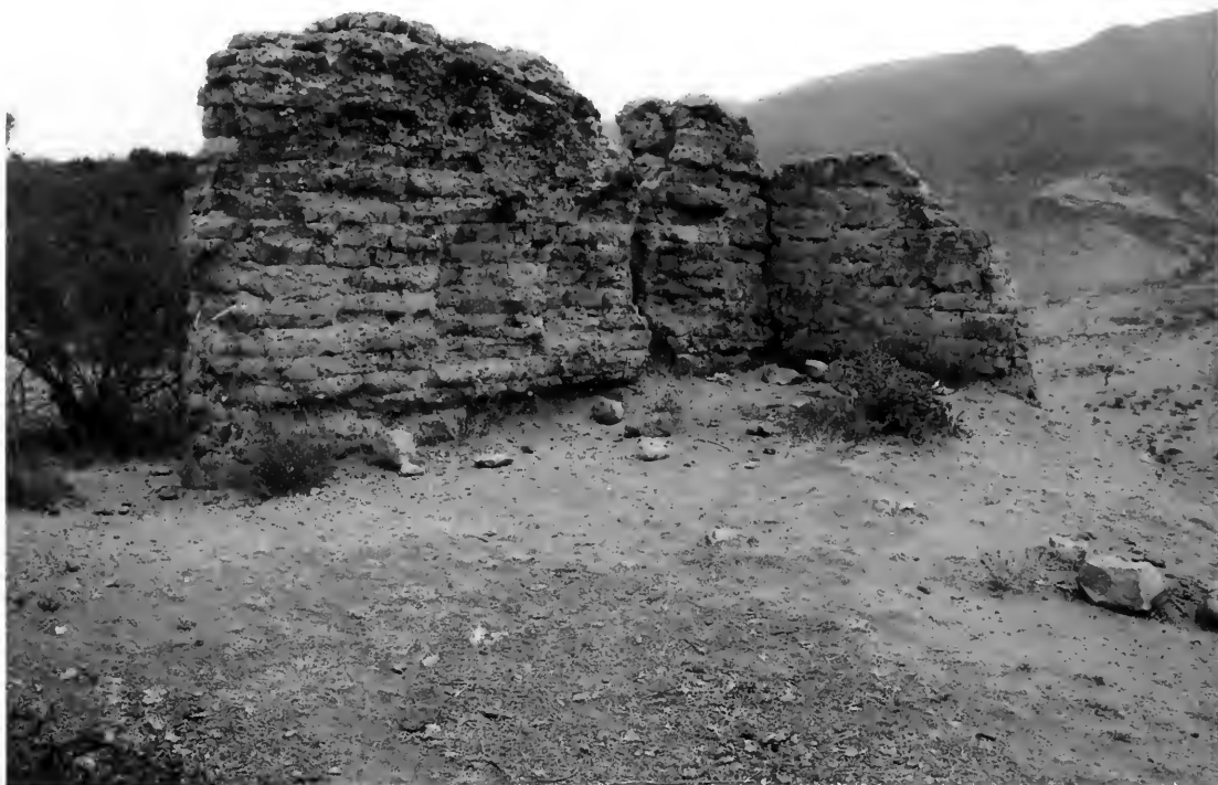
FIG. 3.4. Standing adobe wall (Structure 71) on the summit of the Mitla Fortress.
