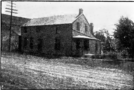
Former residence of Rev. W. H. Collins.
