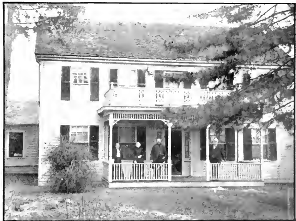
RESIDENCE OF ABRAHAM MCNEILL, SR., Fourth Street
