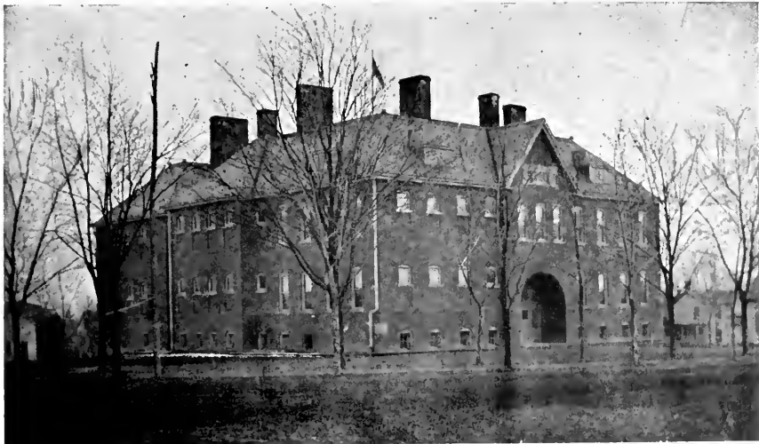
THE GREENVILLE PUBLIC SCHOOL BUILDING, Built in 1894.
