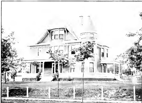
RESIDENCE OF ULYSSES S. DEMOULIN.
