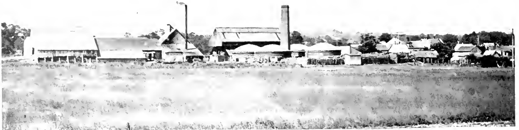
THE PRESSED BRICK PLANT OF THE GREENVILLE LUMBER COMPANY.
