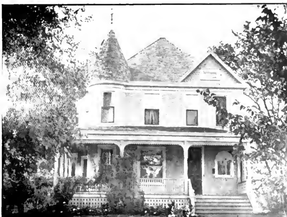
RESIDENCE OF W. D. DONNELL, North Third Street.
