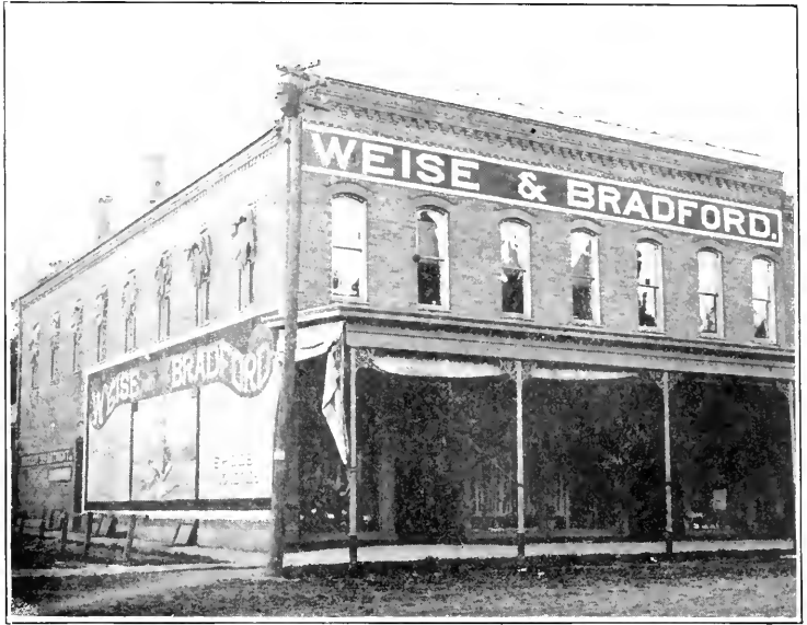
WEISE AND BRADFORD'S GREENVILLE STORE.
