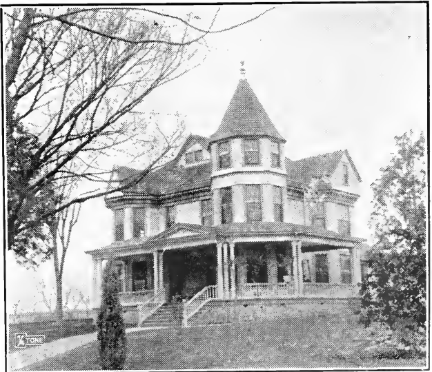
RESIDENCE OF DR. B. F. COOP, West College Avenue.
