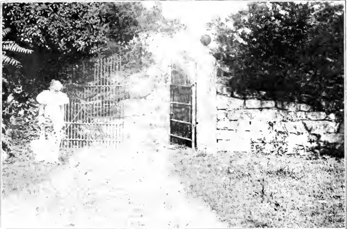
Old Stone Wall and Gateway at Prestwold
