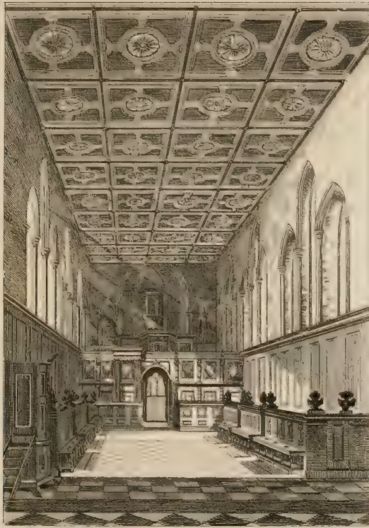
INTERIOR OF THE GREAT HALL
