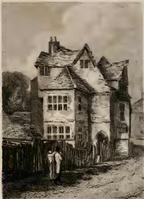
View of the building from the street, showing the entrance and the chimney.
