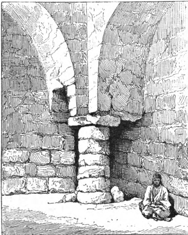
FIG. 85.—Sarvistan. Column and springing of the arches of one of the halls. Ibid. , Plate VI.
