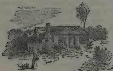
COMMANDANT'S HOUSE, MELBOURNE, 1837.
