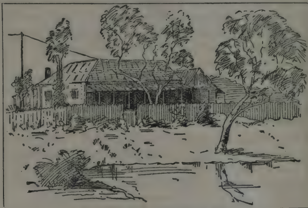
STATION ON OVERLAND TELEGRAPH LINE.
