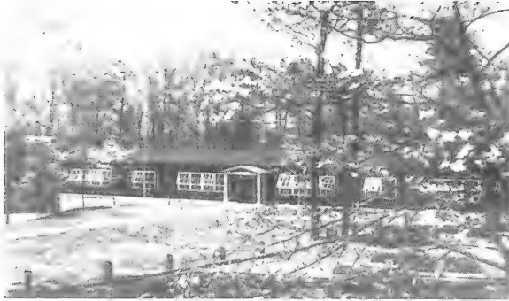
Figure 18. Office and laboratory of the BEB, Washington, D.C., 17 May 1940.
