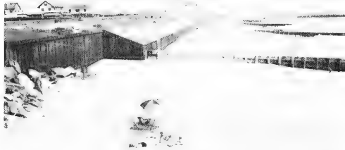
Figure 51. A series of groins and wooden revetments impede recreational use of beach at Deal, New Jersey, 13 August 1936.
