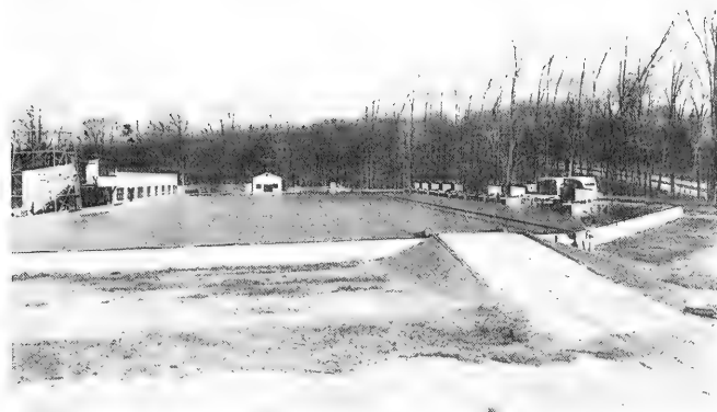
Figure 37. The BEB's shore processes test basin in February 1953. Observation tower on left.
