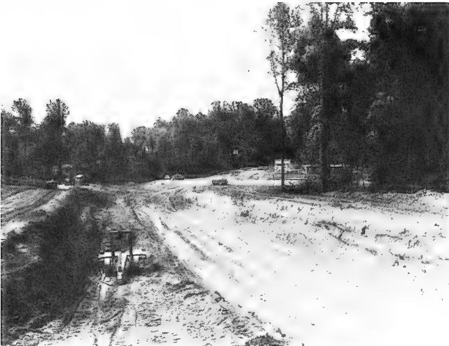
Figure 26. Grading in preparation for the BEB's new 635-foot wave tank, 24 August 1949.
