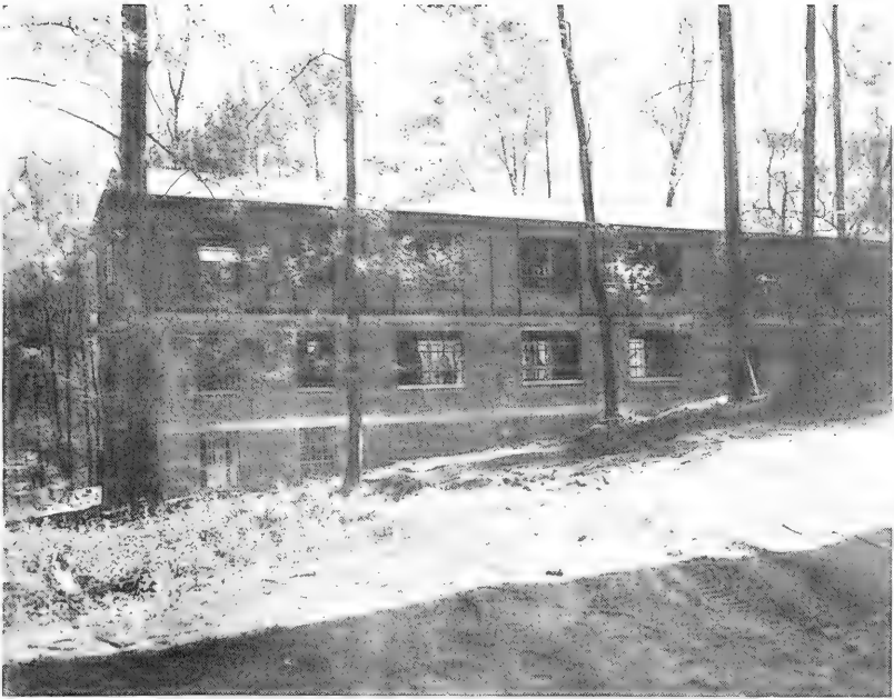
Figure 42. Completed new wing which provided the BEB staff with added office and laboratory space, 1949.
