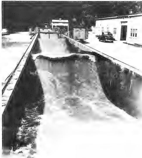
Figure 36. Breaking wave in the BEB's 20-foot-deep, 15-foot-wide, and 635-foot-long wave tank.
