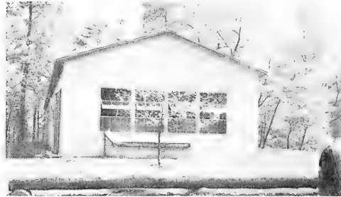
Figure 14. Completed building housing the new 85-foot wave tank of the BEB, located on the Dalecarlia Reservation in Washington, D.C.
