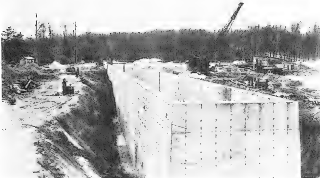
Figure 30. Another view of construction of BEB research facilities, 10 January 1950.
