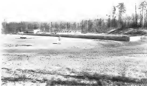
Figure 31. Completed large wave tank but without generator (this was later installed at the far left end of the tank). Shore processes test basin in background.
