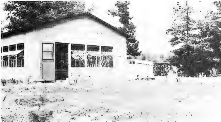
Figure 12. Another view of metal building at Fort Humphreys (later Fort Belvoir), Virginia, housing the BEB's first experimental wave tank.
