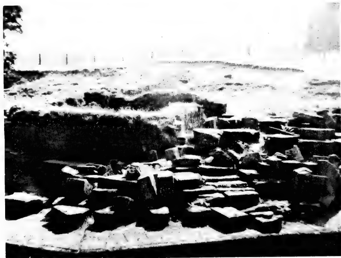
B. Bridge-head showing wall approach and square building.
