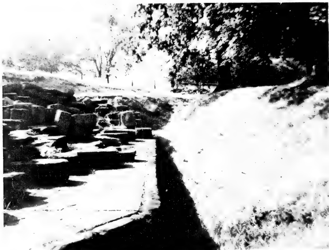
4. Bridge-head showing abutment.
