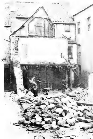
Above. —A mud and straw (“claut and clay”) wall on the northern wall-boundary for 30' in length by 2' thick by 12' high. It was very strong and difficult to demolish. Large stone Tudor fireplace on 1st floor of northern wall, capable of burning 8' logs. Marked X in wall. Roof beams and rafters were of solid rough hewen oak throughout. The lowest room seen here was panelled at a much later date.
