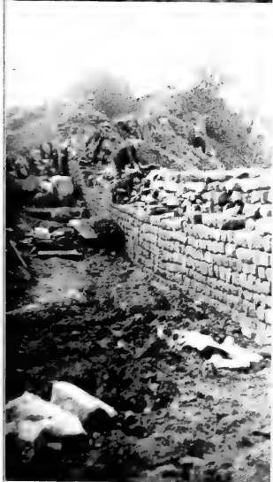
A. North Face of Wall. Note stepped-up foundations.
