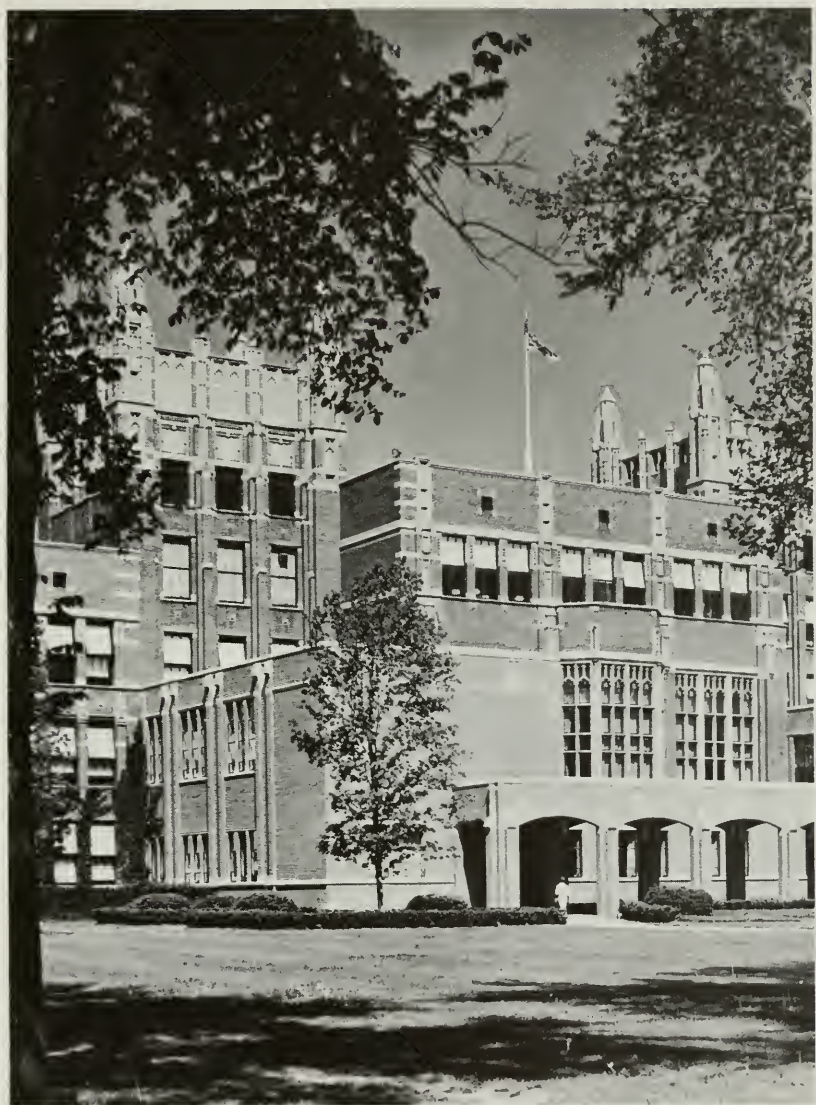
E.T.H.S. today is pictured above with the library and main office additions to the left and right of the Tudor windows, which were part of the original façade of the E.T.H.S. built in 1924.
