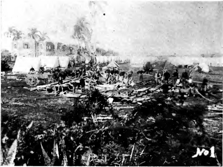
WRECK OF THE TANK.
