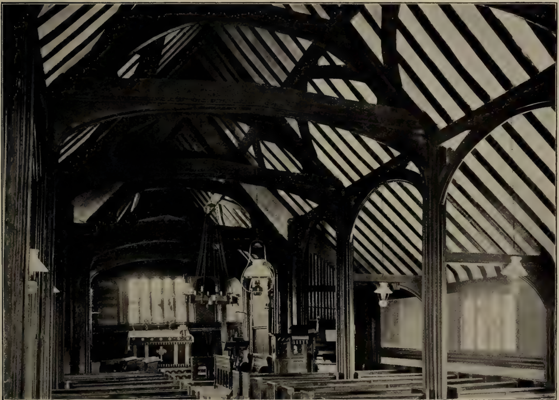
HECKFIELD : MATTINGLEY CHAPEL : THE NAVE LOOKING EAST
