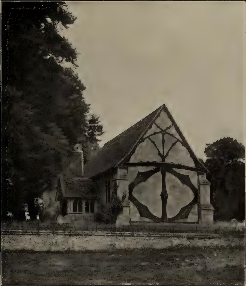
HARTLEY WESPALL CHURCH • WEST END OF NAVE
