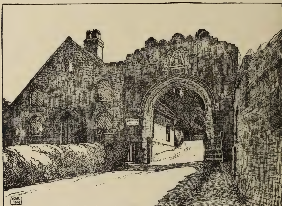
BASING HOUSE GATEWAY.
