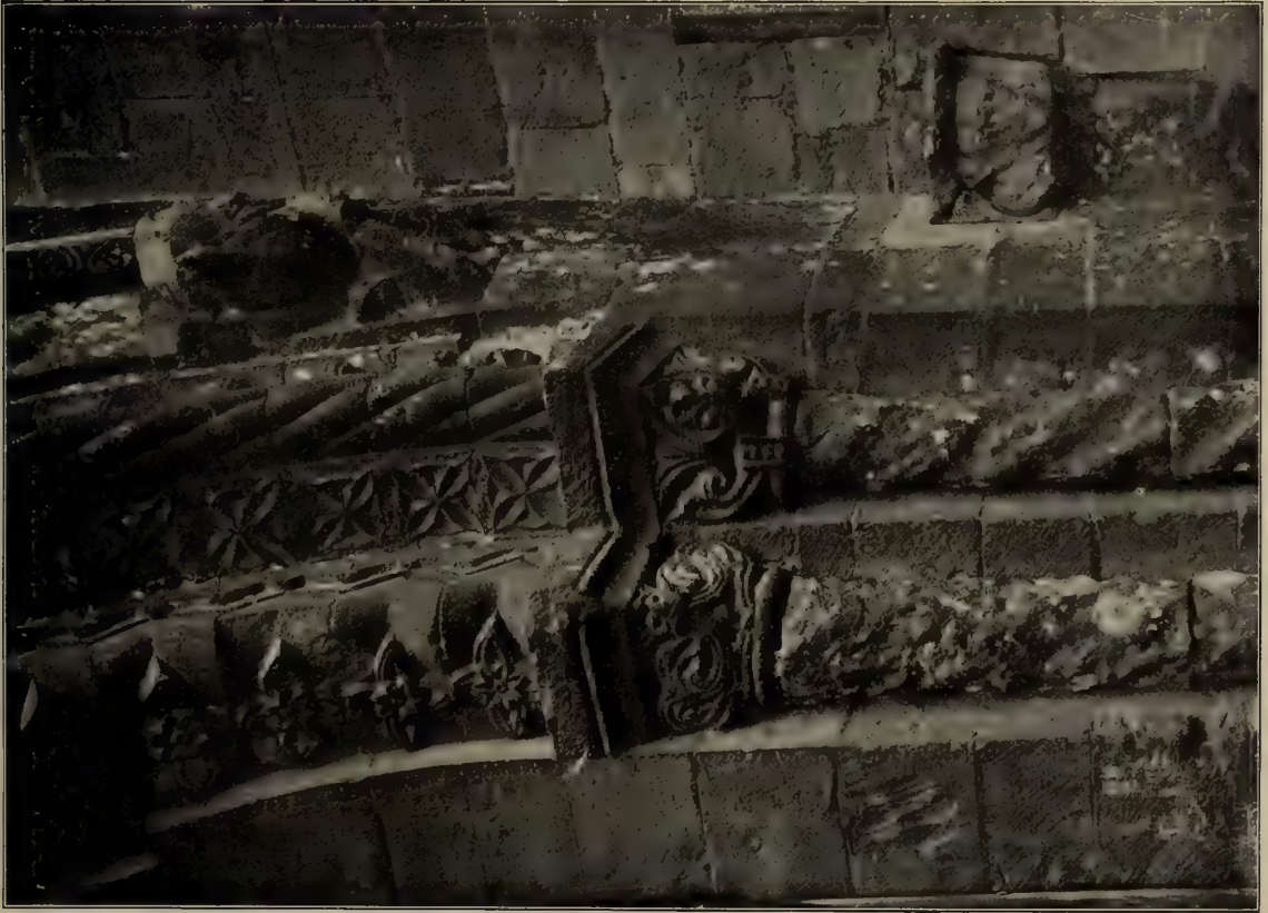
ROMSEY ABBEY : DETAIL OF EAST CLOISTER DOORWAY
