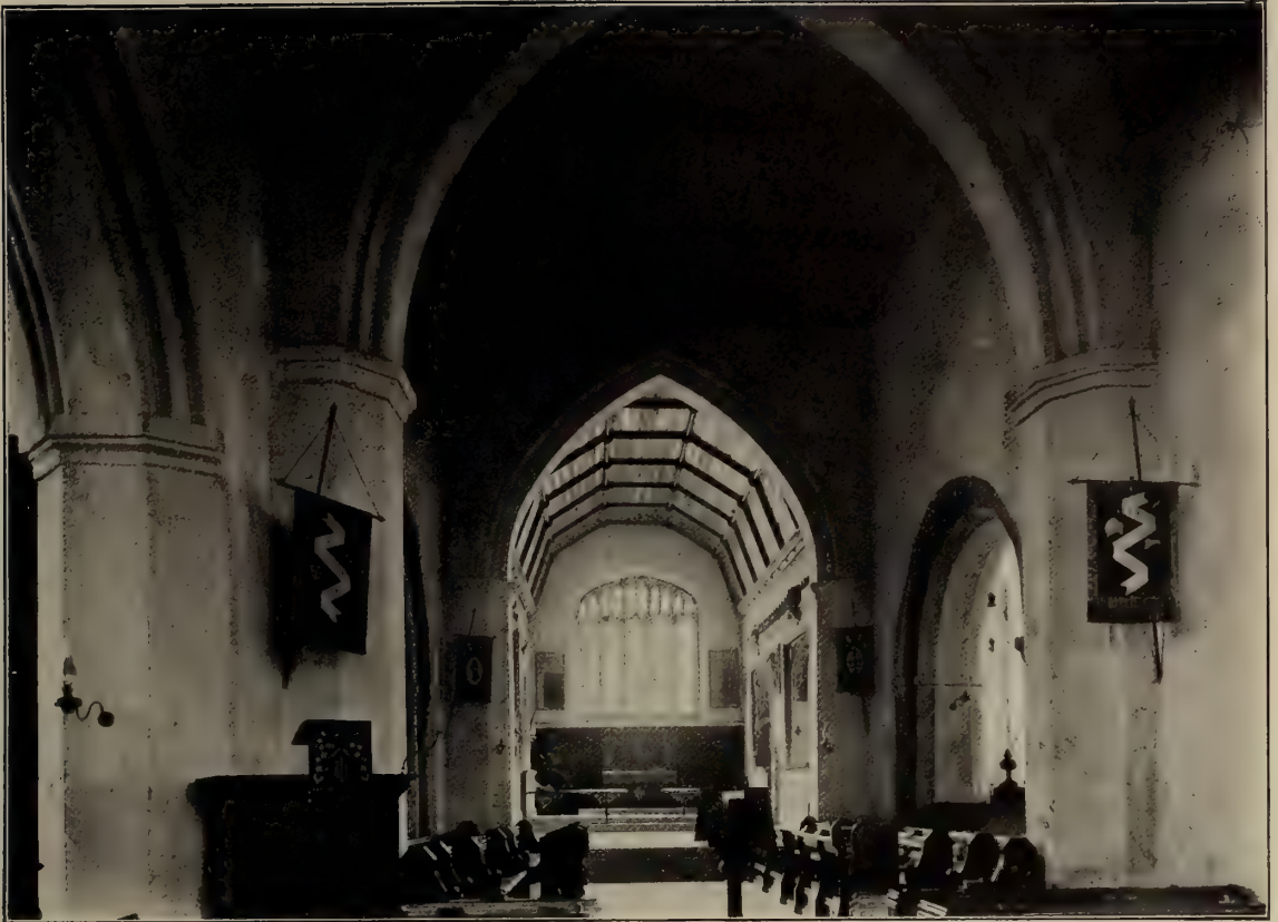
BASING CHURCH : THE NAVE LOOKING EAST
