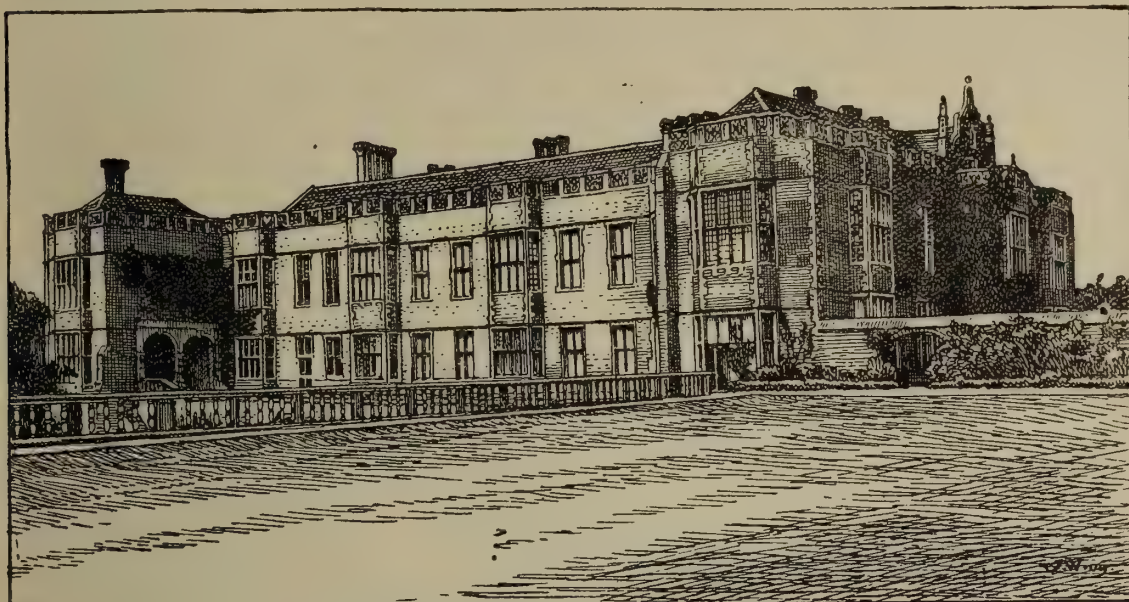
BRAMSHILL HOUSE : SOUTH-EAST FRONT
