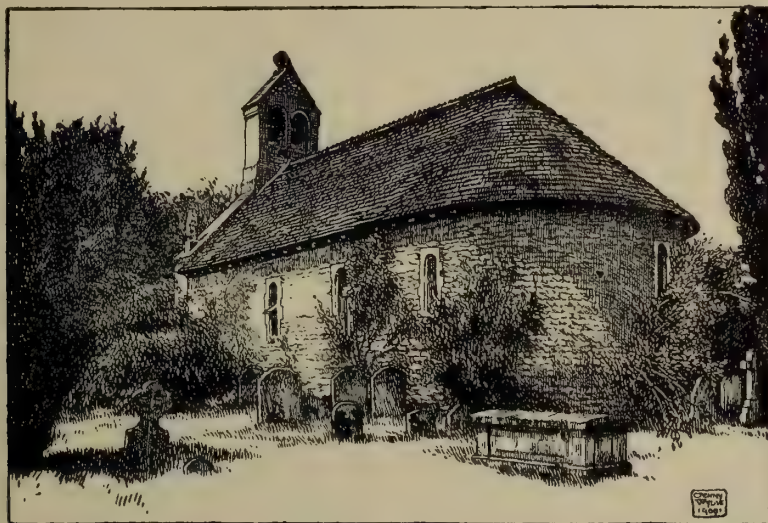
ST. SWITHUN'S CHURCH, NATELY SCURES, FROM SOUTH-EAST
