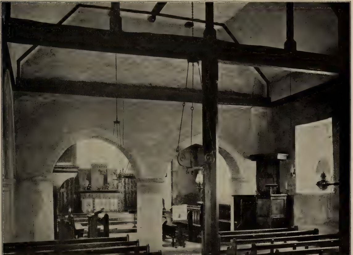
UPPER CLATFORD CHURCH : NAVE LOOKING EAST
