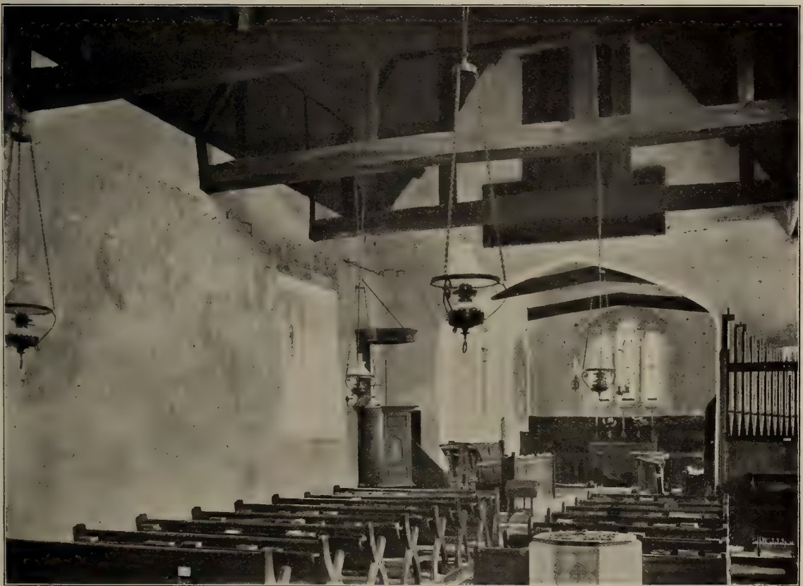
EAST WELLOW CHURCH : NAVE LOOKING EAST
