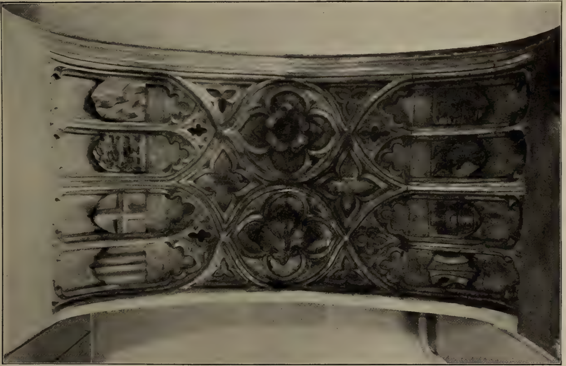
MOTTISFONT PRIORY : SOFFIT OF ARCH OF PULPITUM
