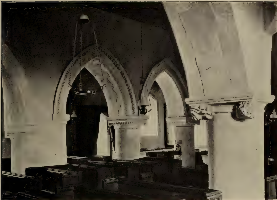
GOODWORTH CLATFORD CHURCH : NAVE LOOKING NORTH-EAST
