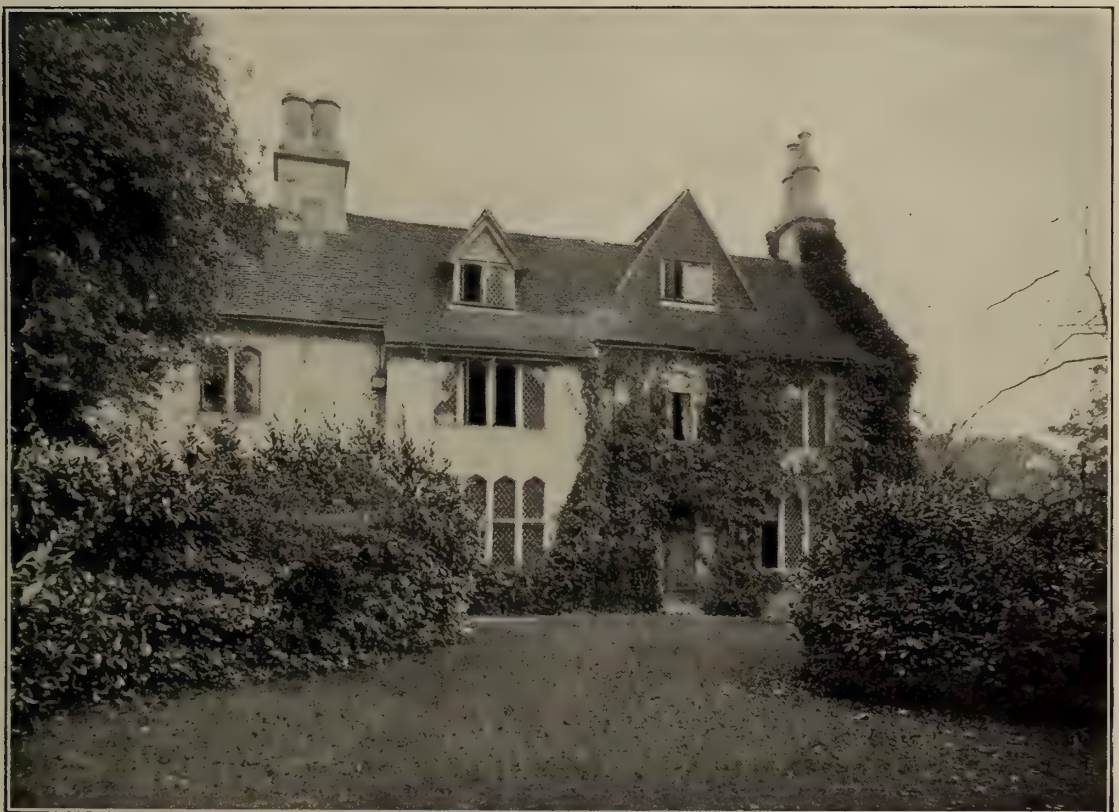
WINCHFIELD RECTORY : WEST FRONT
