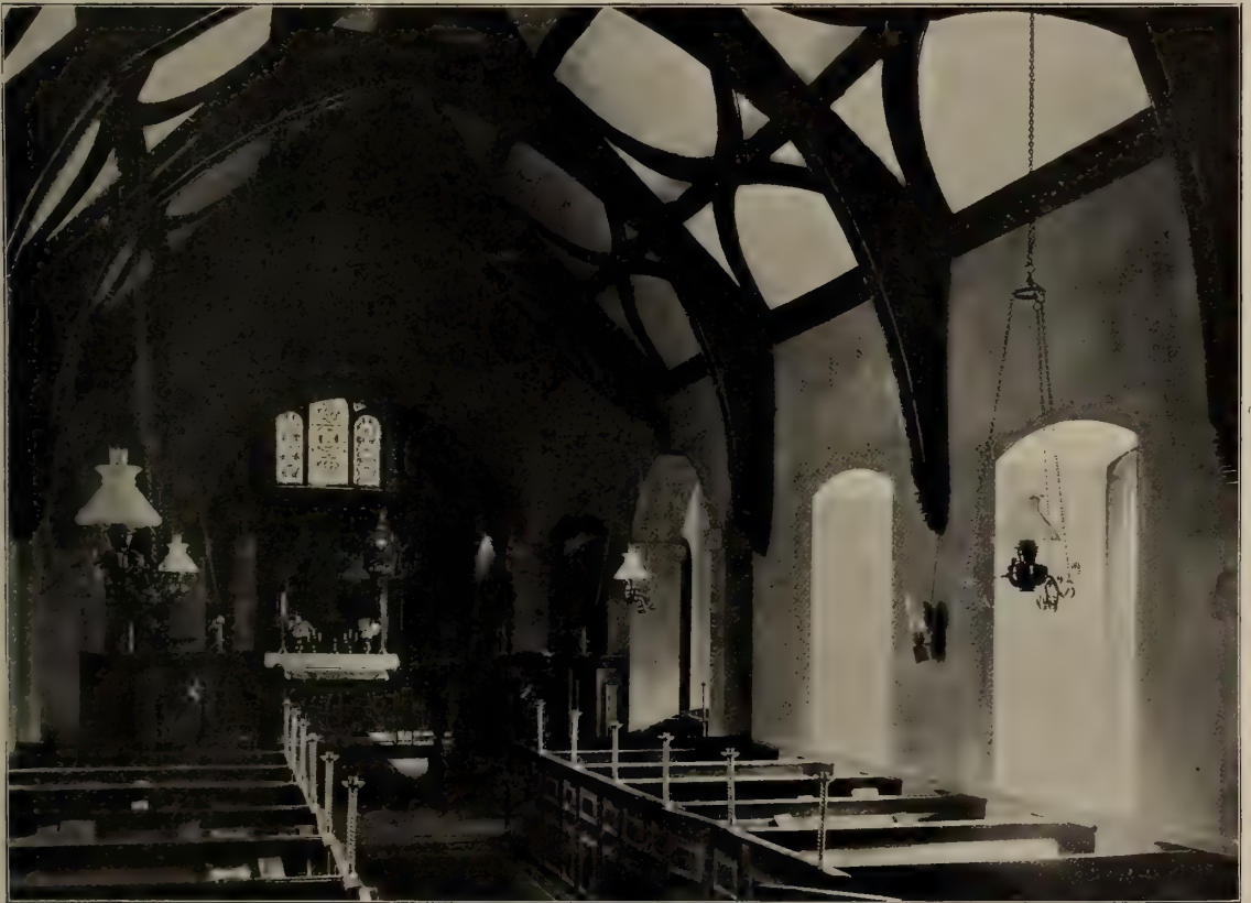
WOLVERTON CHURCH : NAVE LOOKING EAST
