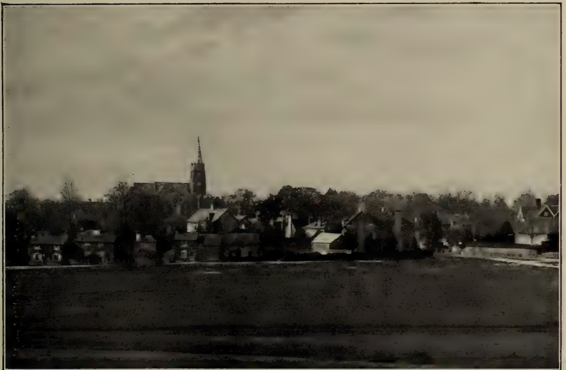
LYNDHURST : GENERAL VIEW FROM THE NORTH
