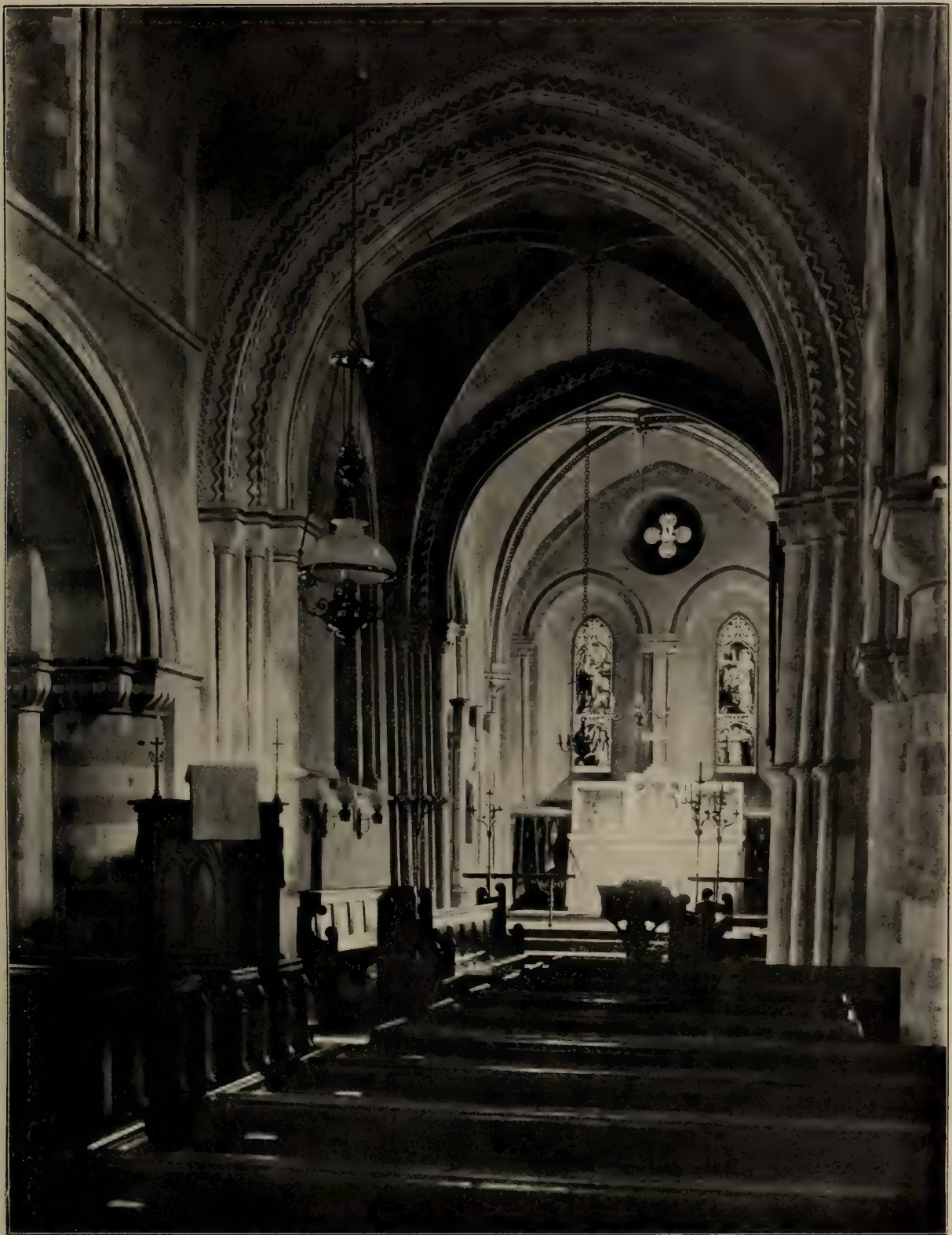
CRONDALL CHURCH : THE NAVE LOOKING EAST
