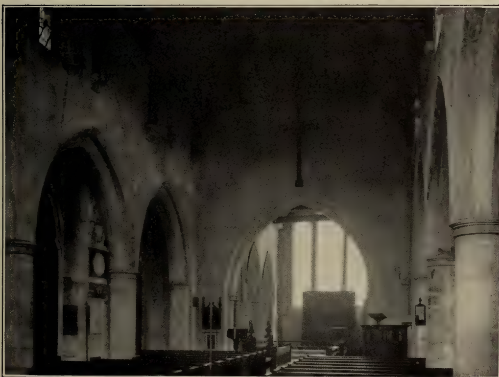
FORDINGBRIDGE CHURCH : THE NAVE LOOKING EAST
