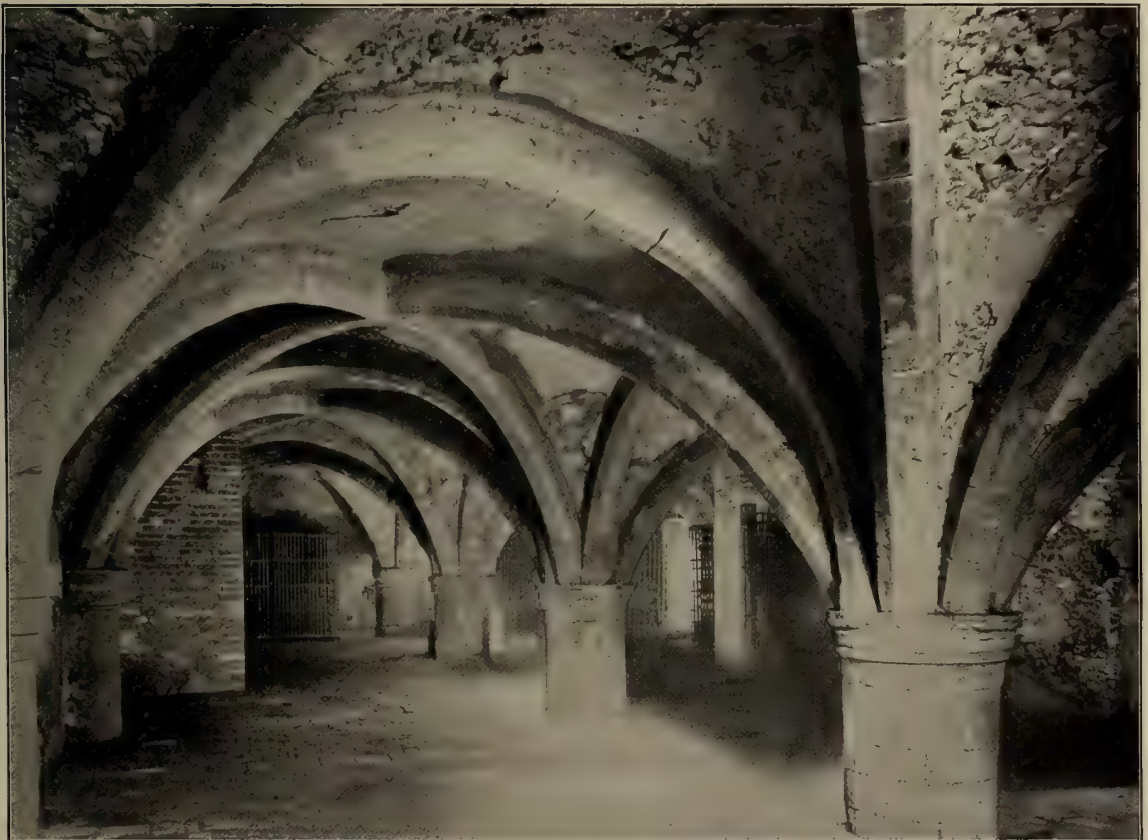
MOTTISFONT PRIORY : SUB-VAULT OF WESTERN RANGE
