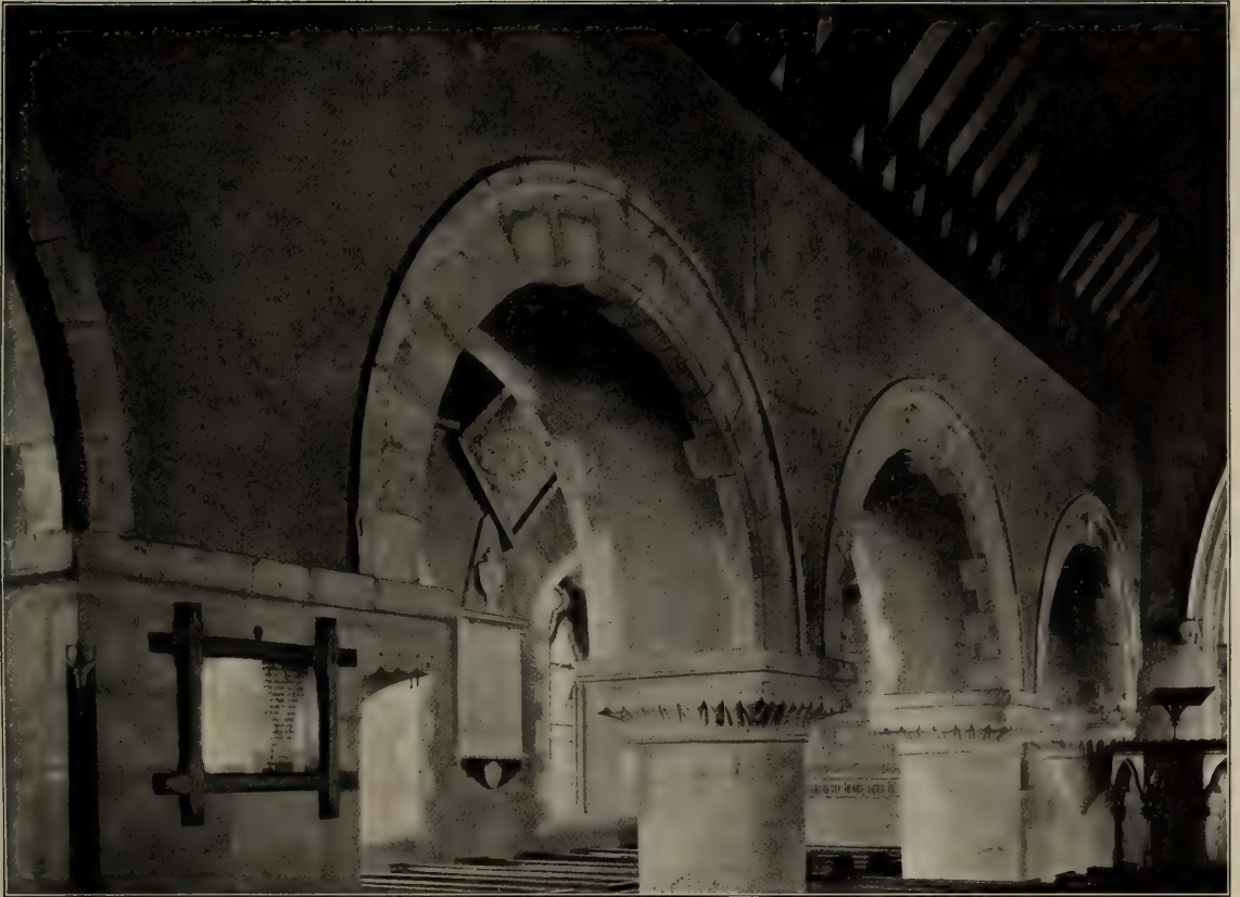
WOOTTON ST. LAWRENCE CHURCH : NORTH ARCADE OF NAVE
