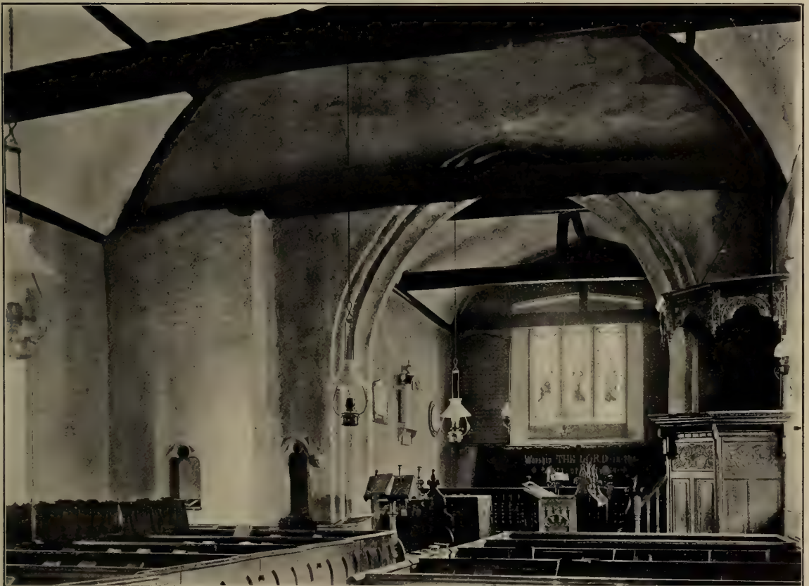
LECKFORD CHURCH : NAVE LOOKING EAST
