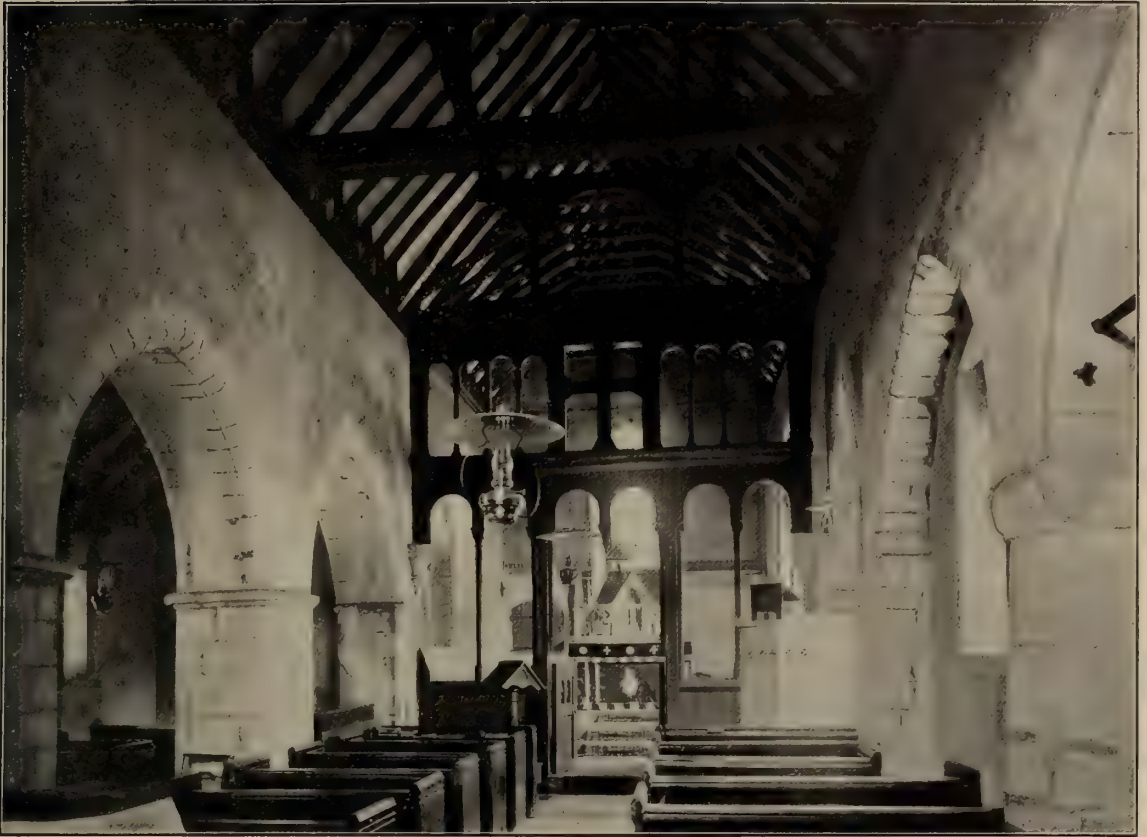
LITCHFIELD CHURCH : NAVE LOOKING EAST
