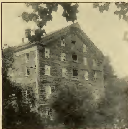
ARTER WAREHOUSE The Only Seven-Story Build- ing in Hanover.
