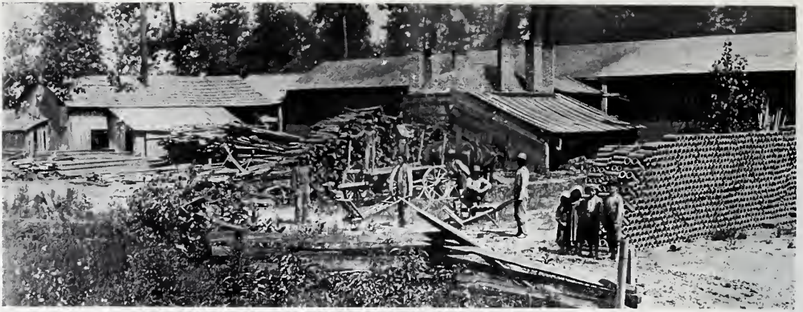
AN OLD VIEW OF THE PLANT
