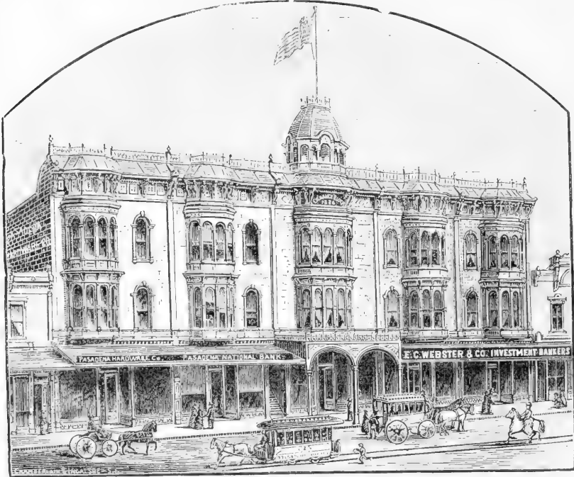
EXCHANGE BLOCK [CARLTON HOTEL], 1866-7.
