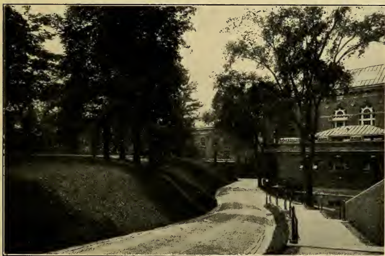
View on Main Roadway
