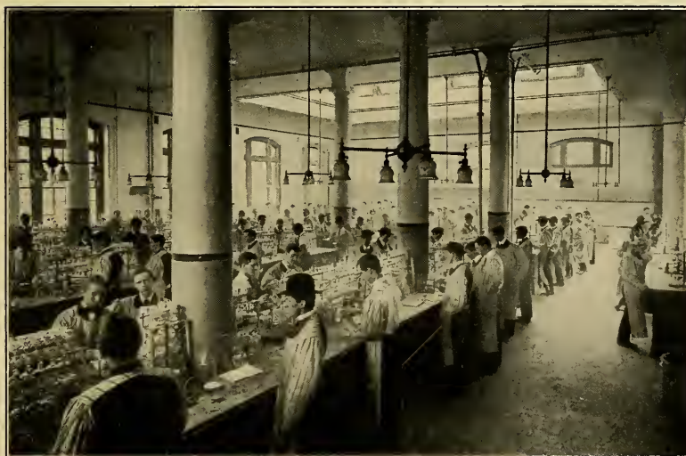
Interior View, Chemical Laboratory
