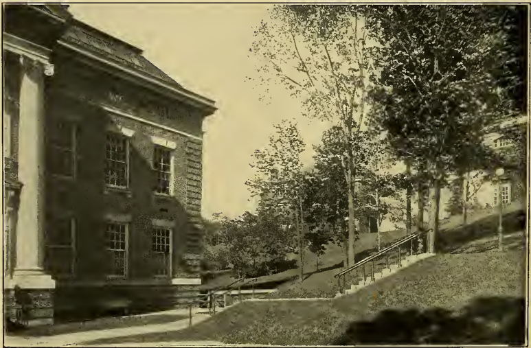
View Southeast of Pittsburgh Building
