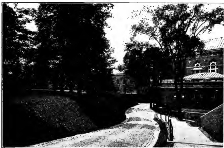
View on Main Roadway
