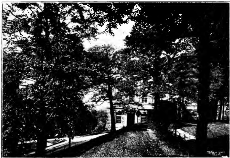
View South of Walker Laboratory
