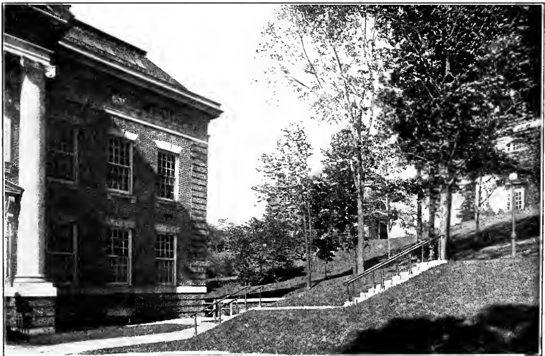
View Southeast of Pittsburgh Building
