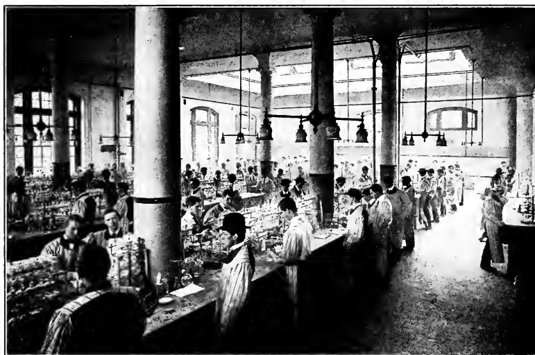
Interior View, Chemical Laboratory
