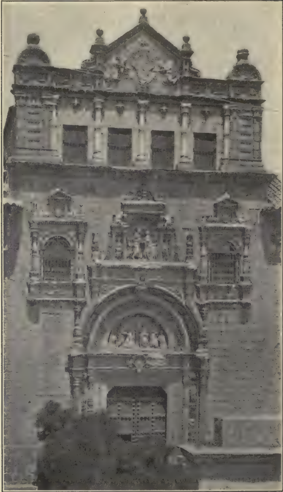
FIGURE 171. — Portal of the Hospital of Santa Cruz. Toledo.
