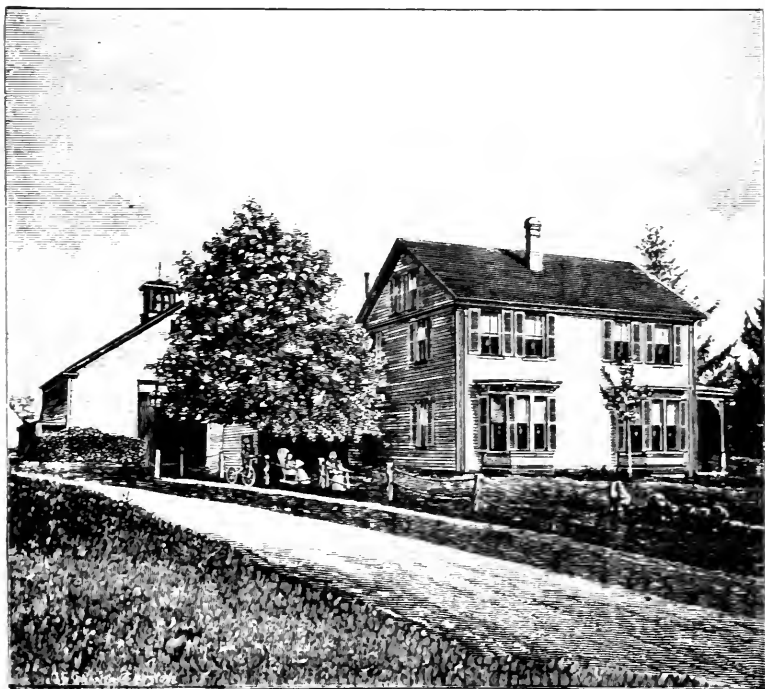
RESIDENCE OF NICHOLS B HUNT, South Sudbury
