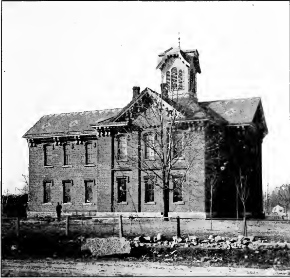
UNIONVILLE SCHOOL BUILDING.
