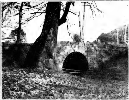
STONE CULVERT BRIDGE ACROSS FINK'S RUN.
