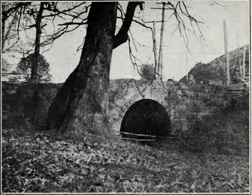
STONE CULVERT BRIDGE ACROSS FINK S RUN.
