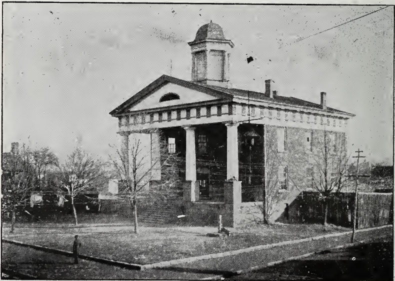
OLD COURT HOUSE.
