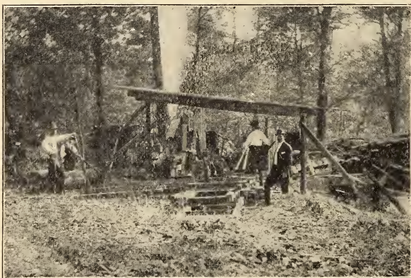
Sawing Lumber on the Campus for Framing for First Building.
