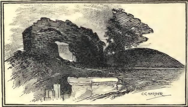
THE "OLD WALL."
