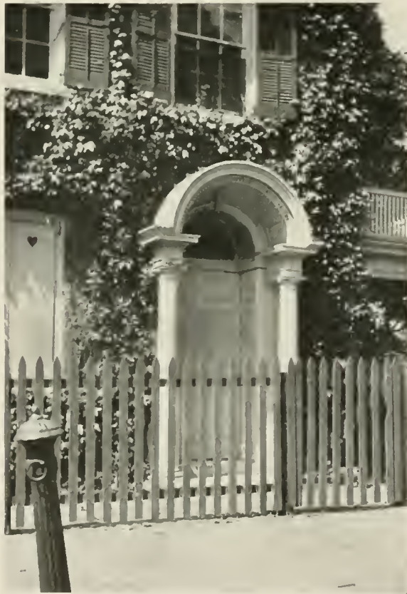
An old hooded doorway at Germantown, Pennsylvania. Note the delicacy of the moldings.
