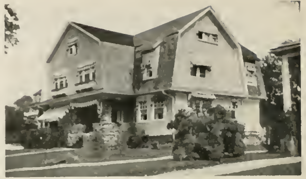
An example of a badly designed gambrel roof. Note the awkward projection of the roof beyond the face of the walls.
