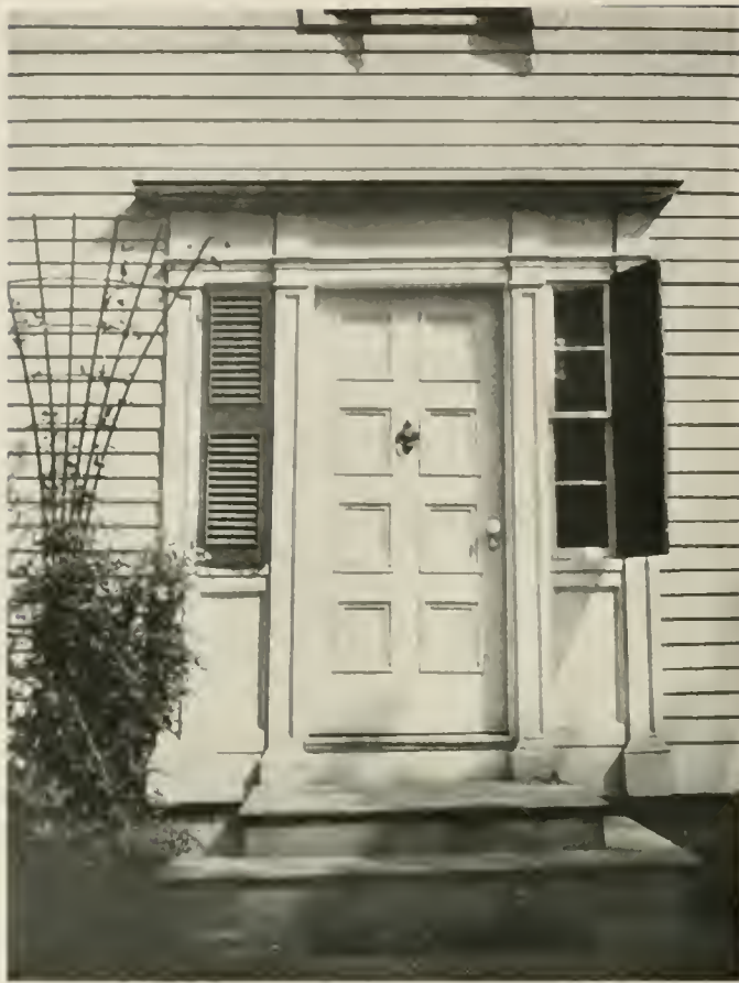
This old doorway which belongs to a house in Pittsfield, Massachusetts, is a fine example of the modest Colonial doorway. The eight panel door and the side lights are characteristic.
