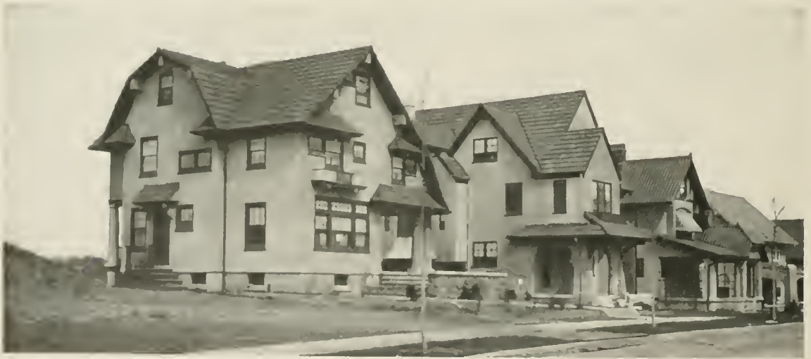
Compare this restless row of badly designed houses with the street of modest white houses on page 61. Compare them also with the group of houses on page 65.
