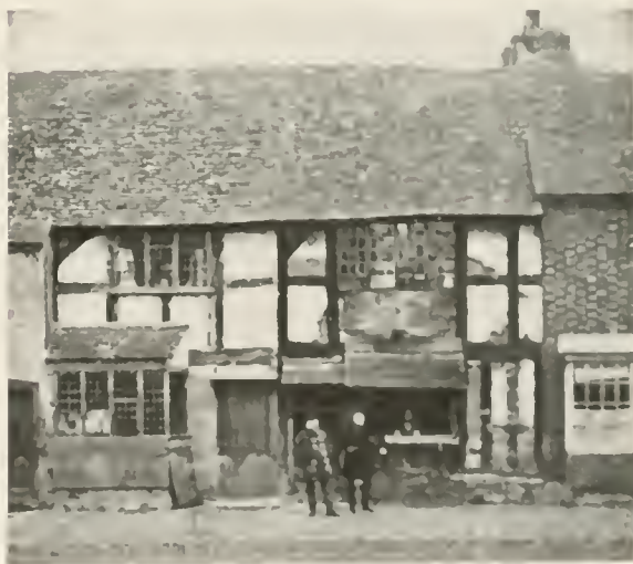
In this old English house, the timber work expresses the actual frame construction of the house.
