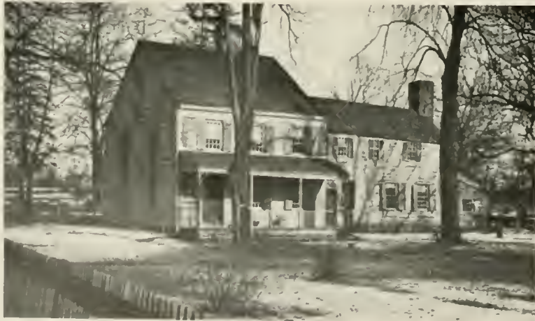
When this attractive old house at Hartsdale, New York, was built, there was a plentiful supply of shingles of good quality. They were more durable than the shingles you can buy nowadays.
