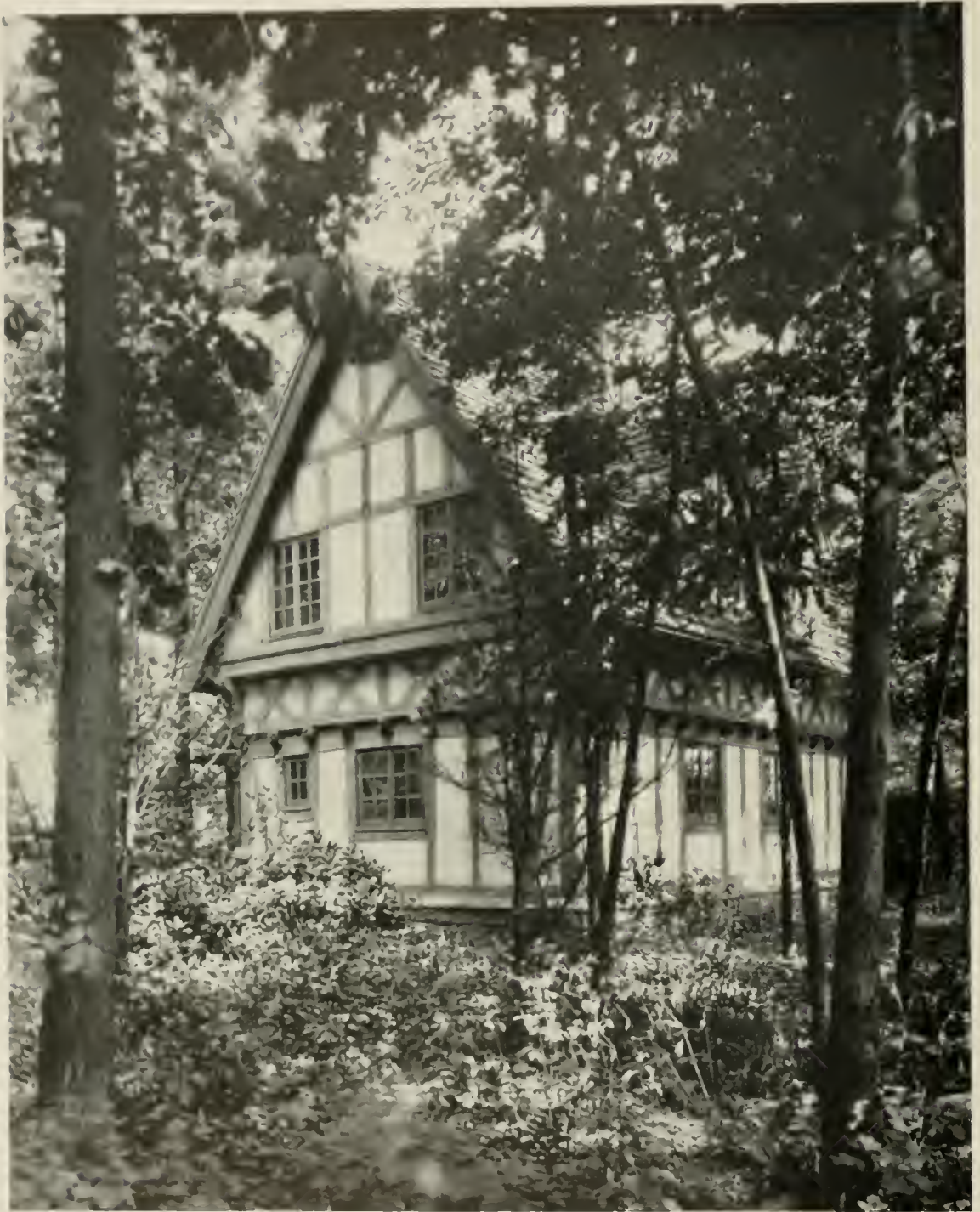
The Vanderbilt Gate Lodge, Deepdale, Long Island.
