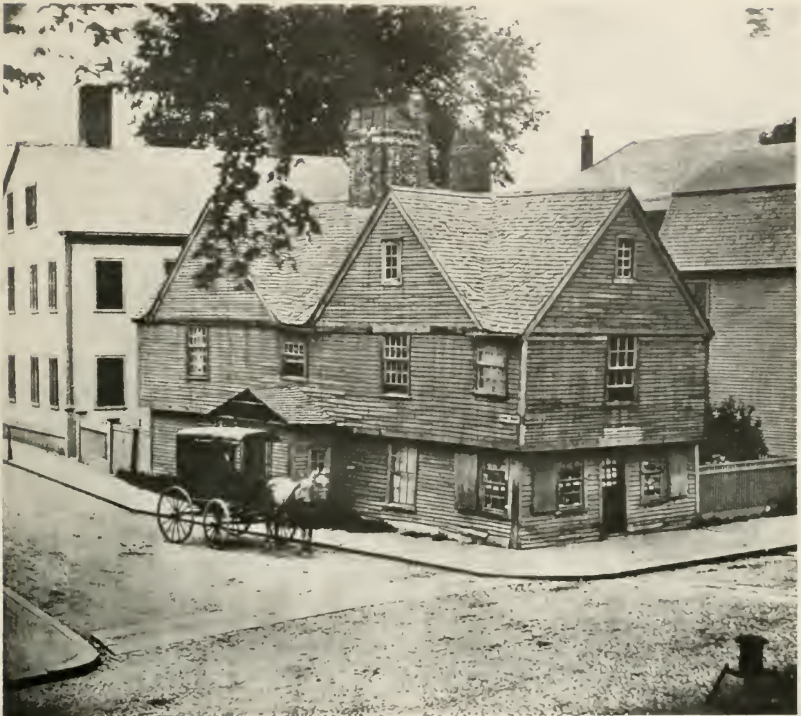
This old gabled house of Salem, Massachusetts, shows beautifully the English architecture of the seventeenth century, transplanted in America. Its gables, its projecting second story and its huge chimney, can still be seen in the old English villages, only the materials, owing to local conditions, are somewhat different.
