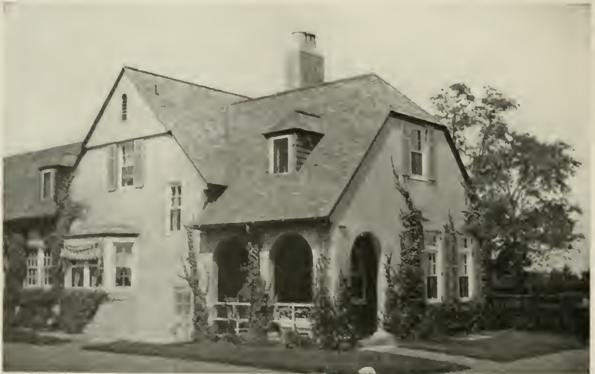
Howard Greenley, Architect. The small arcaded porch of the gardener's cottage on Mr. C. A. Coffin's estate at Locust Valley, Long Island, is full of charm. The roof which is cut off on the gable end might better have terminated in the usual way.
