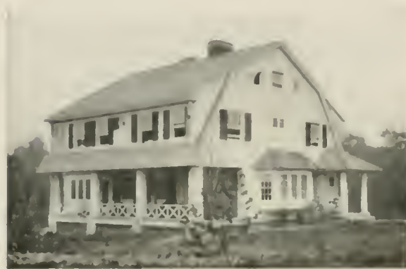
Another illustration of bad roof lines. If the dormer has to be so big, why try to have a gambrel roof?
