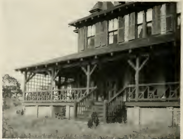
This represents the idea of a seaside cottage as the architect of 1880 conceived it. Note the ugly posts and the fantastic railing.
