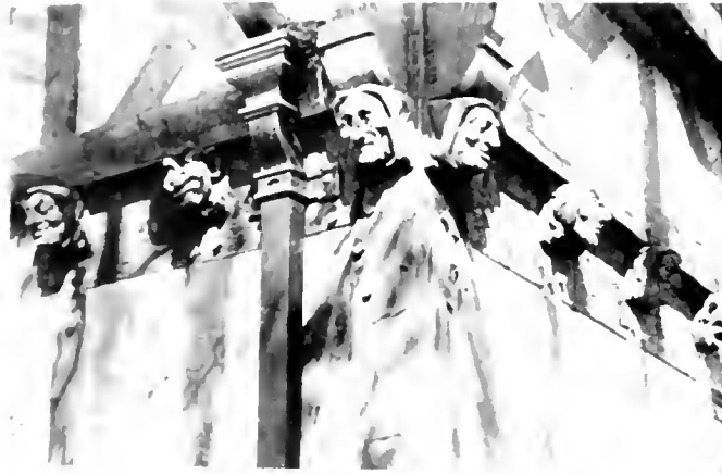
John Russell Pope, Architect. A detail of the Vanderbilt Lodge at "Deepdale" showing the carved gargoyles.
