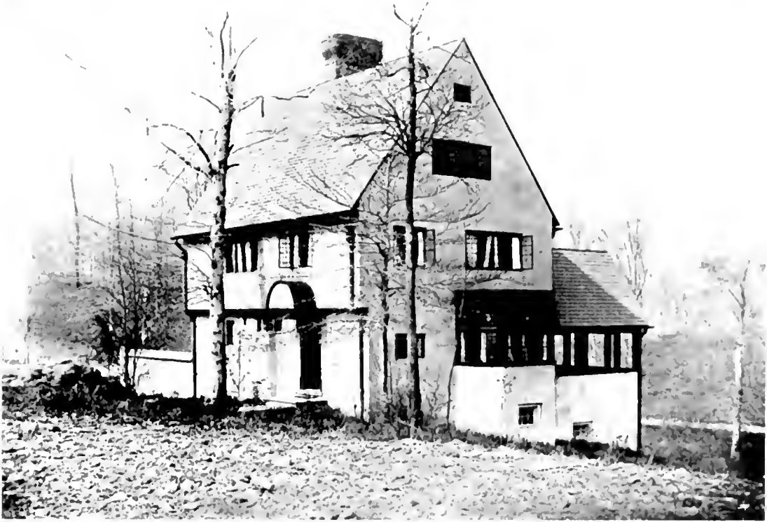
Mr. Dow's house at Summit, New Jersey, is full of unusual detail. Note the leaded glass windows, the plain, steep roof, the strong contrast between the stained woodwork and the stucco walls. Joy Wheeler Dow, Architect.
