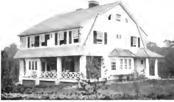
Another illustration of bad roof lines. If the dormer has to be so big, why try to have a gambrel roof?
