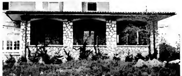
This shows how not to build a stone wall.
