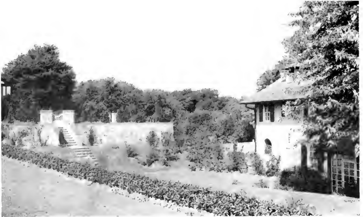
Edmund B. Gilchrist, Architect. This shows the advantages of a well-arranged foreground. The house is Mr. W. W. Gilchrist's at St. Martins, Philadelphia.
