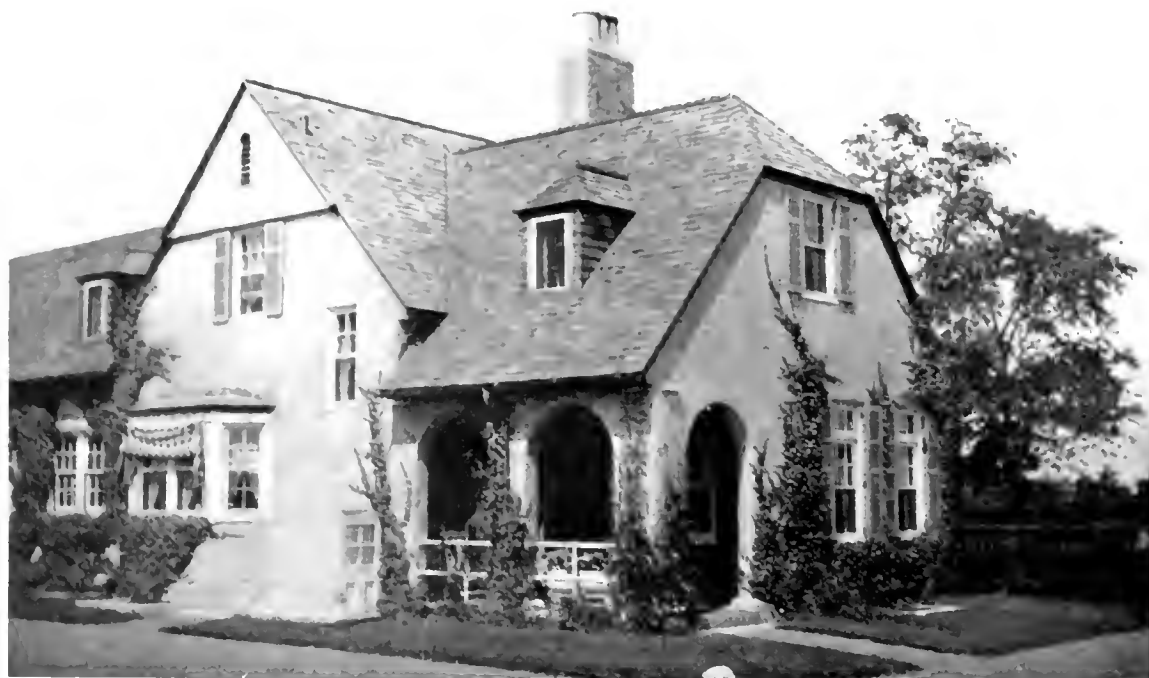
Howard Greenley, Architect. The small arcaded porch of the gardener's cottage on Mr. C. A. Coffin's estate at Locust Valley, Long Island, is full of charm. The roof which is cut off on the gable end might better have terminated in the usual way.
