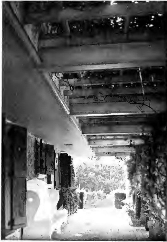
Charles Barton Keen, Architect. Note the unusual arrangement of beams in this pergola porch.
