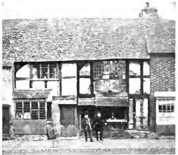
In this old English house the timber work expresses the actual frame construction of the house.
