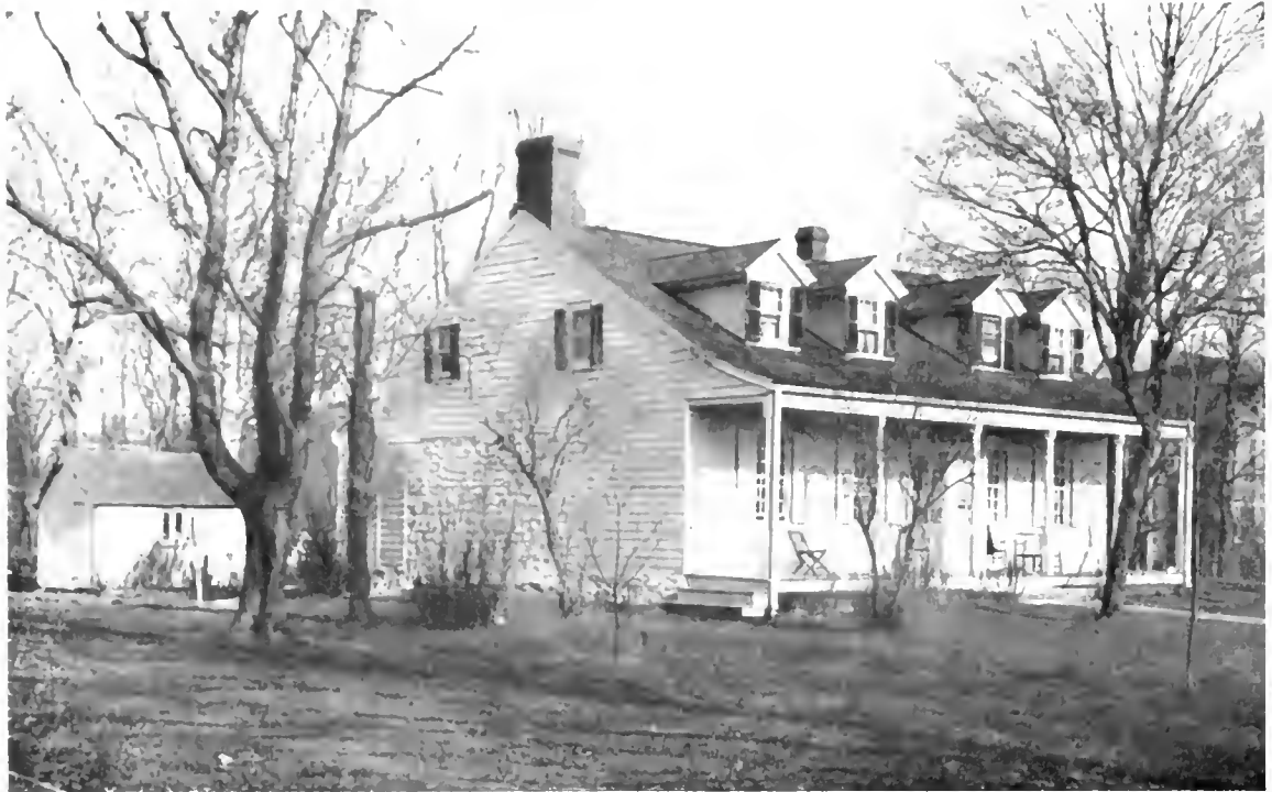
The sunlit porch of this old house at Mt. Vernon, New York, is very inviting.
