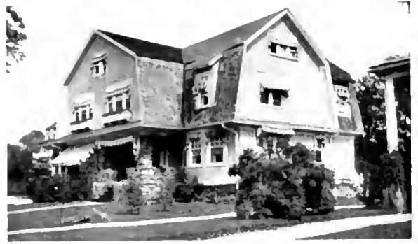
An example of a badly designed gambrel roof. Note the awkward projection of the roof beyond the face of the walls.
