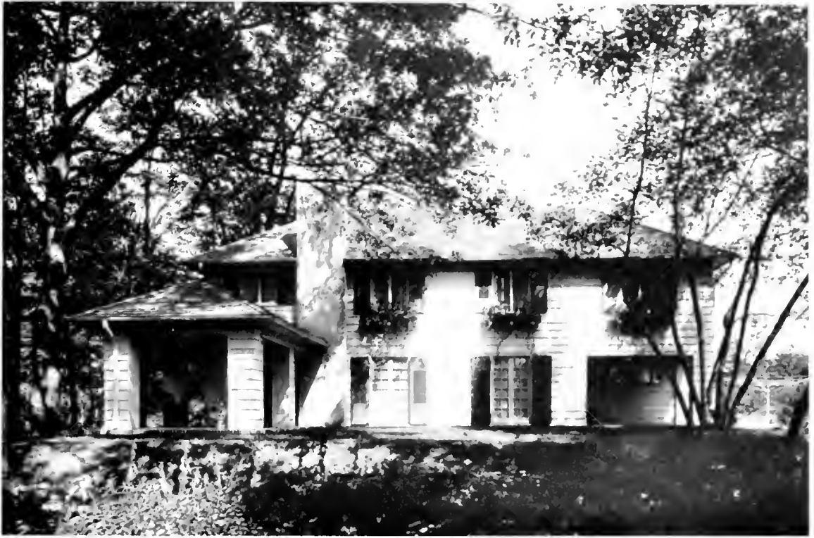
Eugene J. Lang, Architect In Mr. Lang's house at Scarsdale, New York, broad clapboards are employed. The placing of the windows under the long roof, and the general horizontal expression of all the details, gives the house a low-lying quality.
