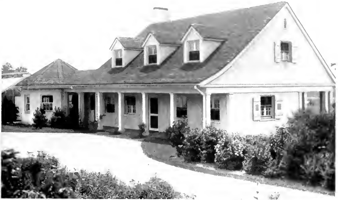
H. Van Buren Magomigle, Architect. The Gardener's Lodge on the estate of Franklin Murphy, Wendham, New Jersey. The design of this house, which in general is excellent, would be improved, perhaps, by the omission of the horizontal band on the gable end.
