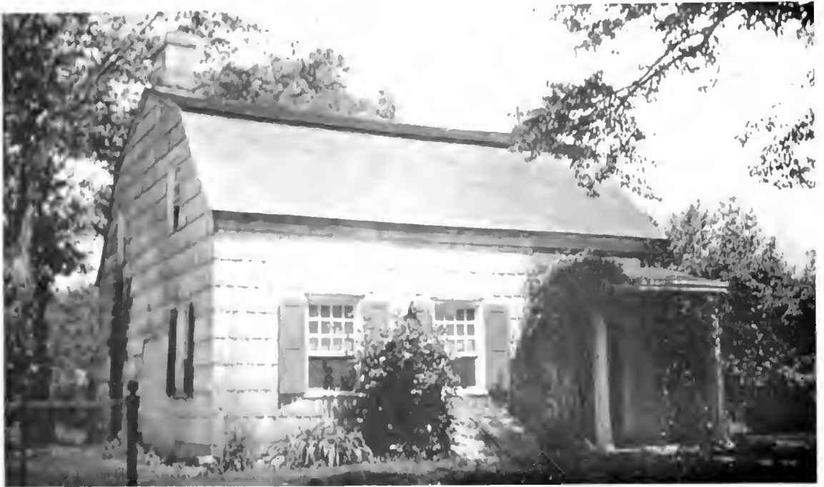
A little house at Garden City, Long Island, that has survived many generations of fashions in house-building. It will always be good,—because it always was. The long hand-split shingles are characteristic of early Long Island work.
