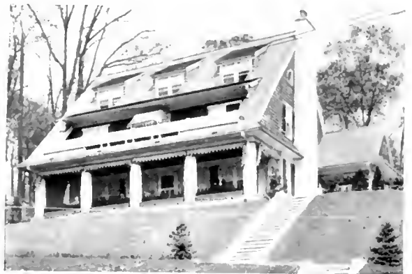
What a roof ought not to look like.
