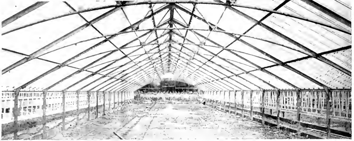
This house of P. S. Randolph's Sons, at Verona, Pa., is 30 feet wide and 175 feet long. Note the arch truss.
