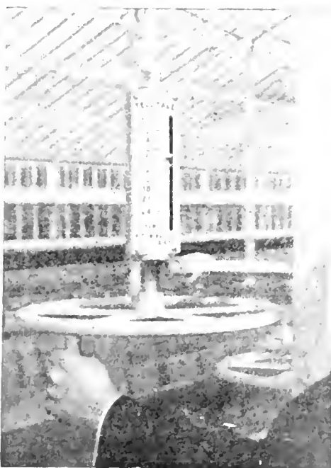
New Tell Tale device. It records in inches the exact opening of your ridge sash.
