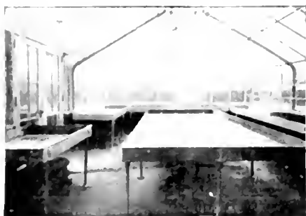
Glimpse of the greenhouse interior, looking towards the fine light gable. The benches have galvanized cast iron sides and bottoms. Every bit of iron and steel in the house is galvanized and aluminum finished.
