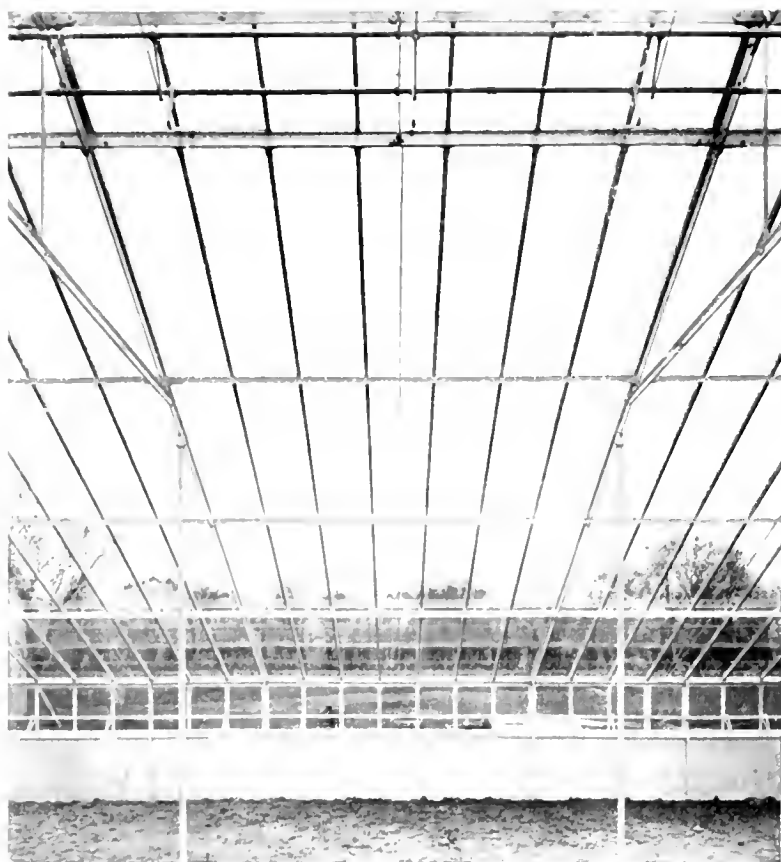
Side view in one of our Reconstructed Constructions, erected for L. B. Coddington, Murray Hill, N. J. Being only 78 feet wide the framing is exceedingly simple and surprisingly light in effect.
