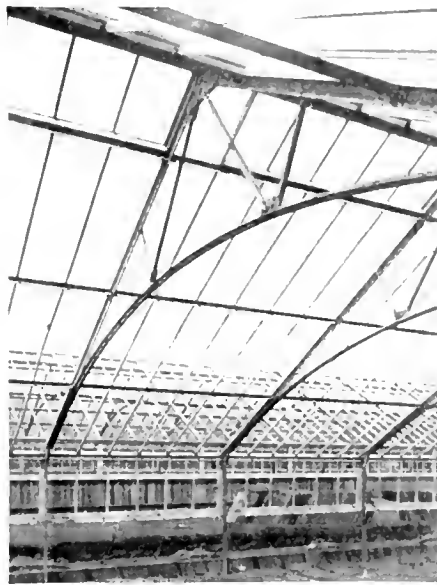
The double angle irons of the arch start at the eave on both sides of the rafter, and for 3 feet or so are bolted directly to it.
