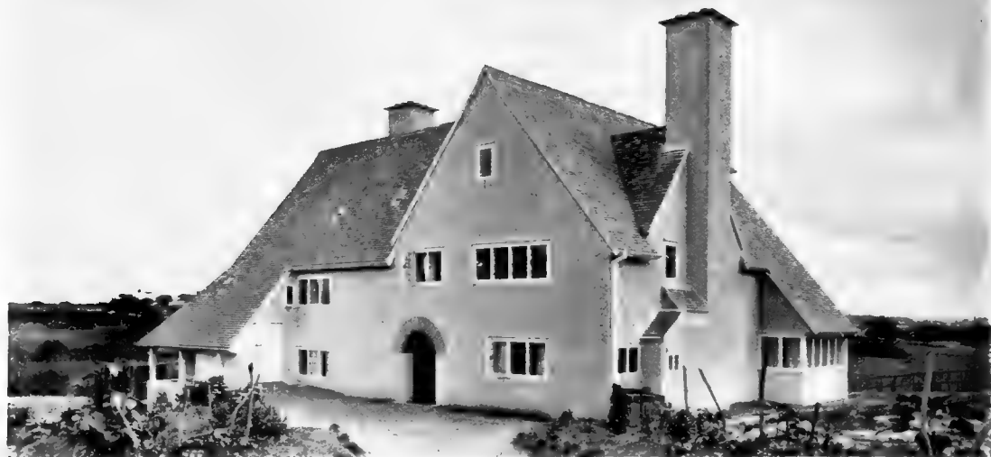
VIEW FROM NORTH-EAST
