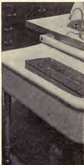
FIG. 26.—Porcelain sink, showing sink strainer and goose-neck faucet. Such an outfit is especially good for the laboratory; also for pantry.
