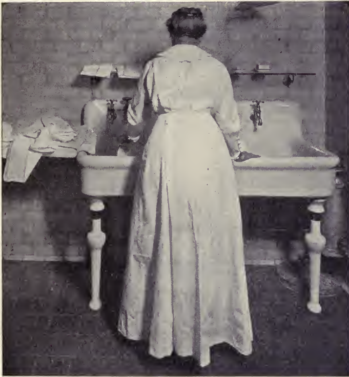
FIG. 31.—This shows the bracelet extension which may be used to raise all low sinks. This sink is divided to furnish a place for washing and rinsing dishes.
