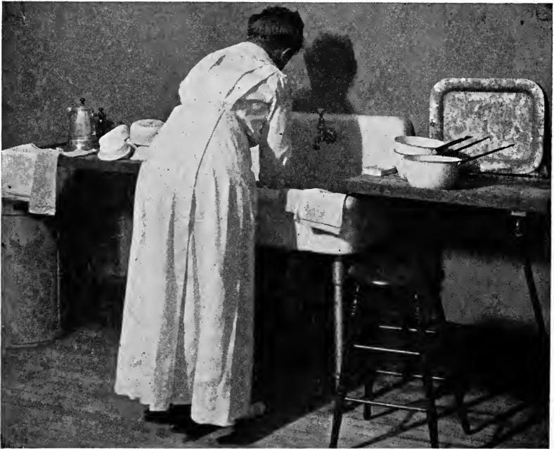
FIG. 30.—Sink only 50 per cent. efficient, because it is set too low for the worker. The standard of sink materials and drainboards good.
