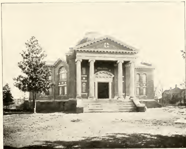
THE NEW CHURCH
