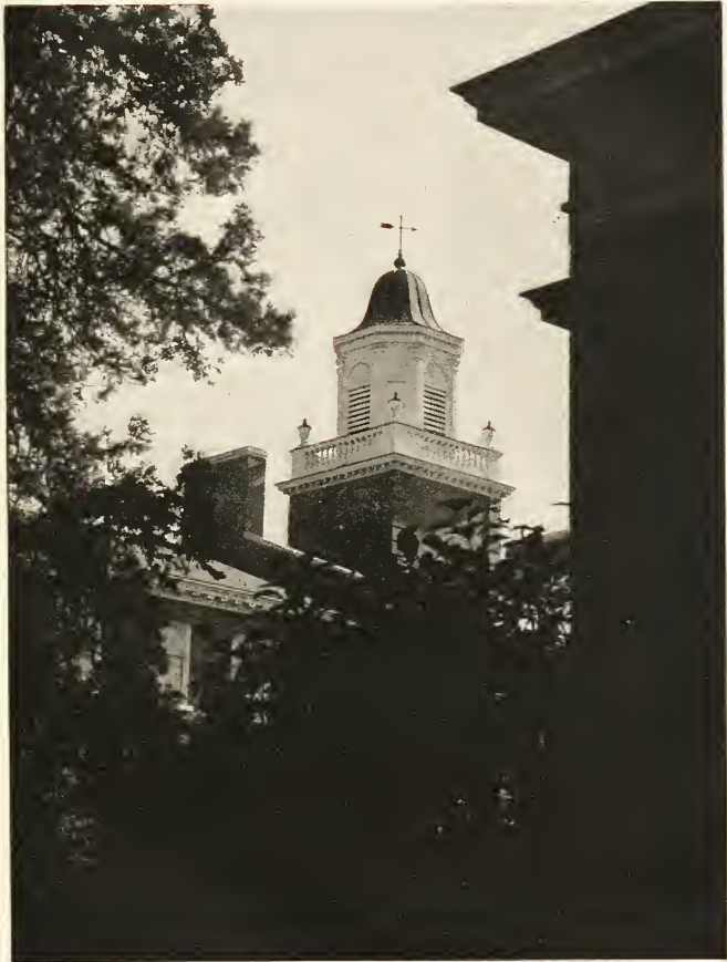
Bell Tower, West Hall
